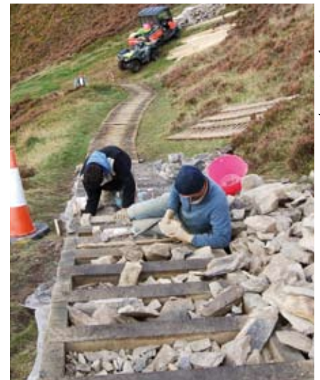
The construction of the floating ramp to protect the slopes of Moel Fenlli
