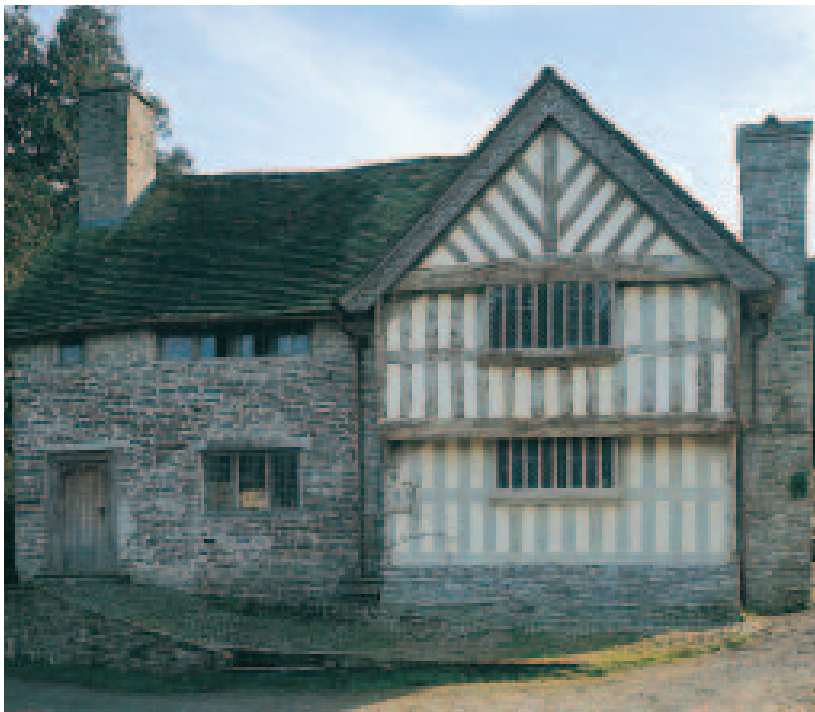
Upper House, Discoed, is listed Grade II*. This timber-framed hall-house was built in the sixteenth century and remodelled in the seventeenth century.
