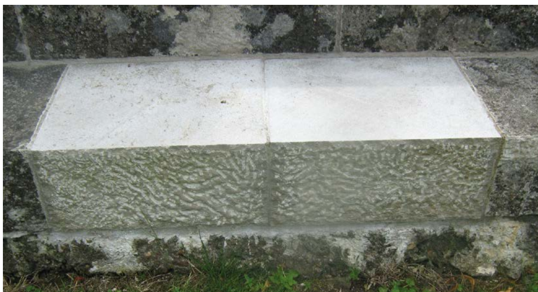
When stone replacement is essential, the new stone should be dressed to match the original. In this example from St Fagans, the top surface is smooth and the facing edge has been rusticated to match the stone alongside (© War Memorials Trust).
