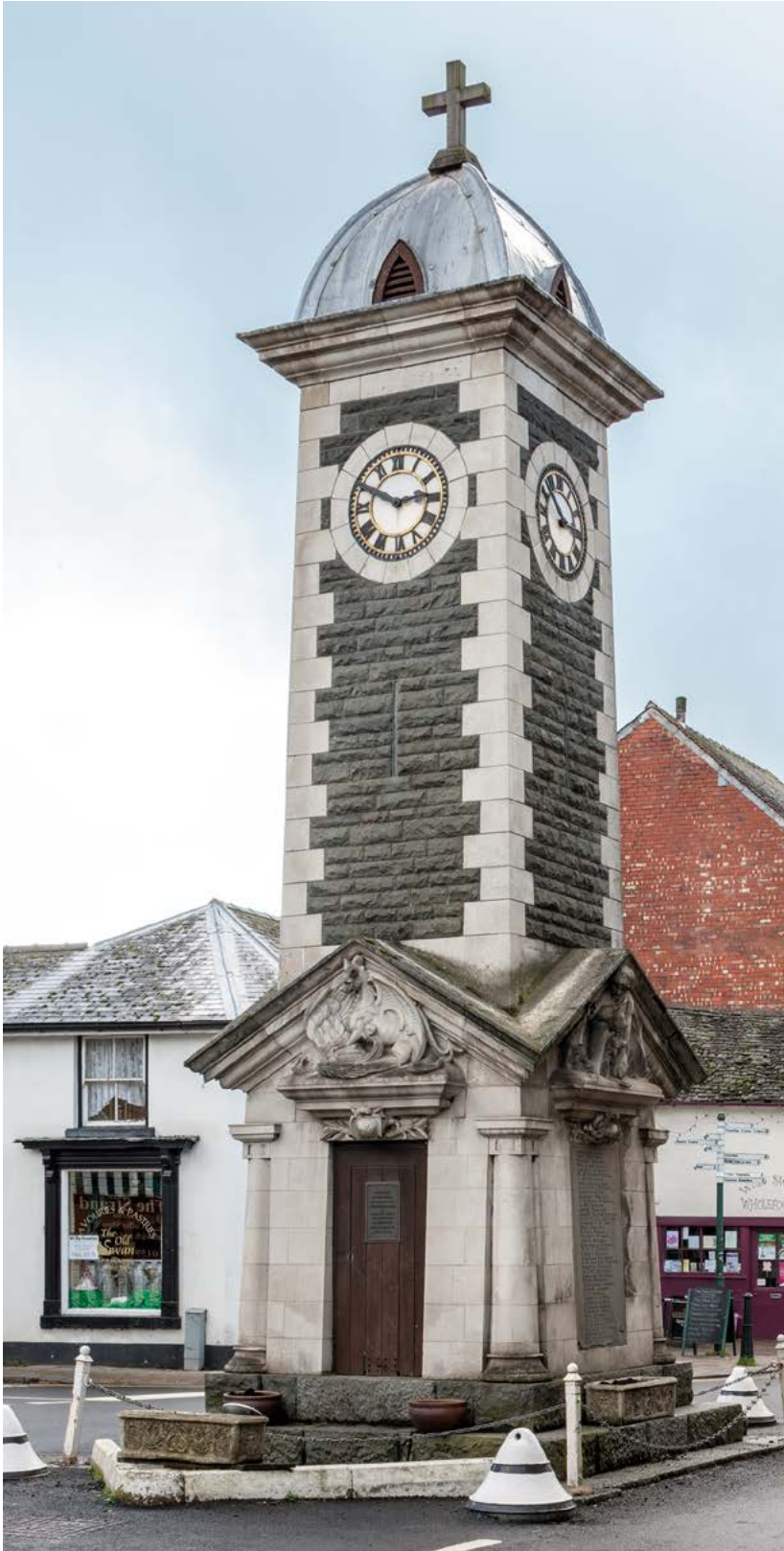
War memorials vulnerable to damage from passing traffic can be protected by bollards. The low bollards around the war memorial at Rhayader protect the monument, but pose little risk to traffic.
