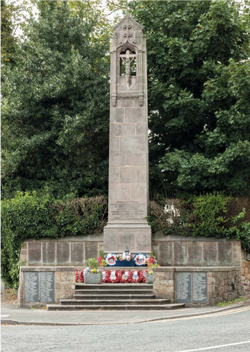
Left: A good photographic record is important. This view shows the Hawarden memorial in context, including the panels which have been added to commemorate the Second World War.
