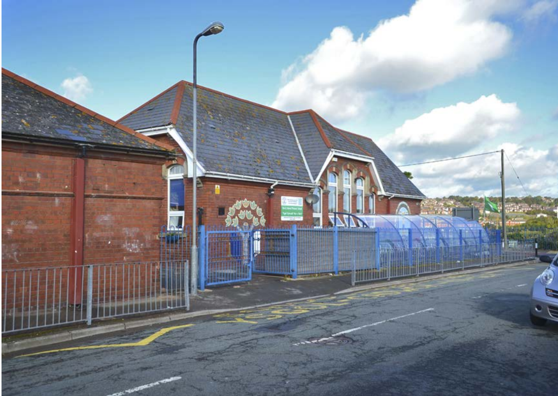
Left: The Archer Road elevation of Barry Island Primary School. Photographed in 2011 (© Civic Trust Cymru).
