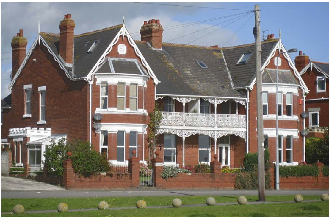
18 and 20 are more ornate with decorative ironwork balconies. Photographed in September 2011 (© Civic Trust Cymru).
