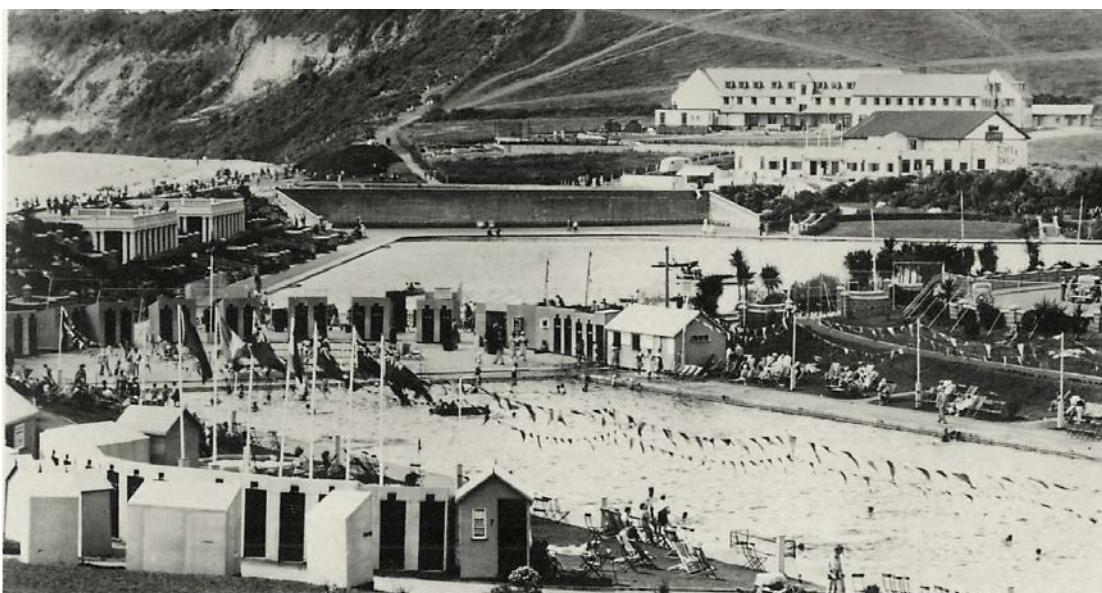
An interwar view of the public works at Cold Knap, Barry. The scheme included the remodelling of the seaside resort on Barry Island. The lido was opened in 1926. The Glanymor YMCA conference and holiday centre in the background was built in 1931–33 and demolished in 1980 (TuckDB Postcards, BRY 3, not dated).
