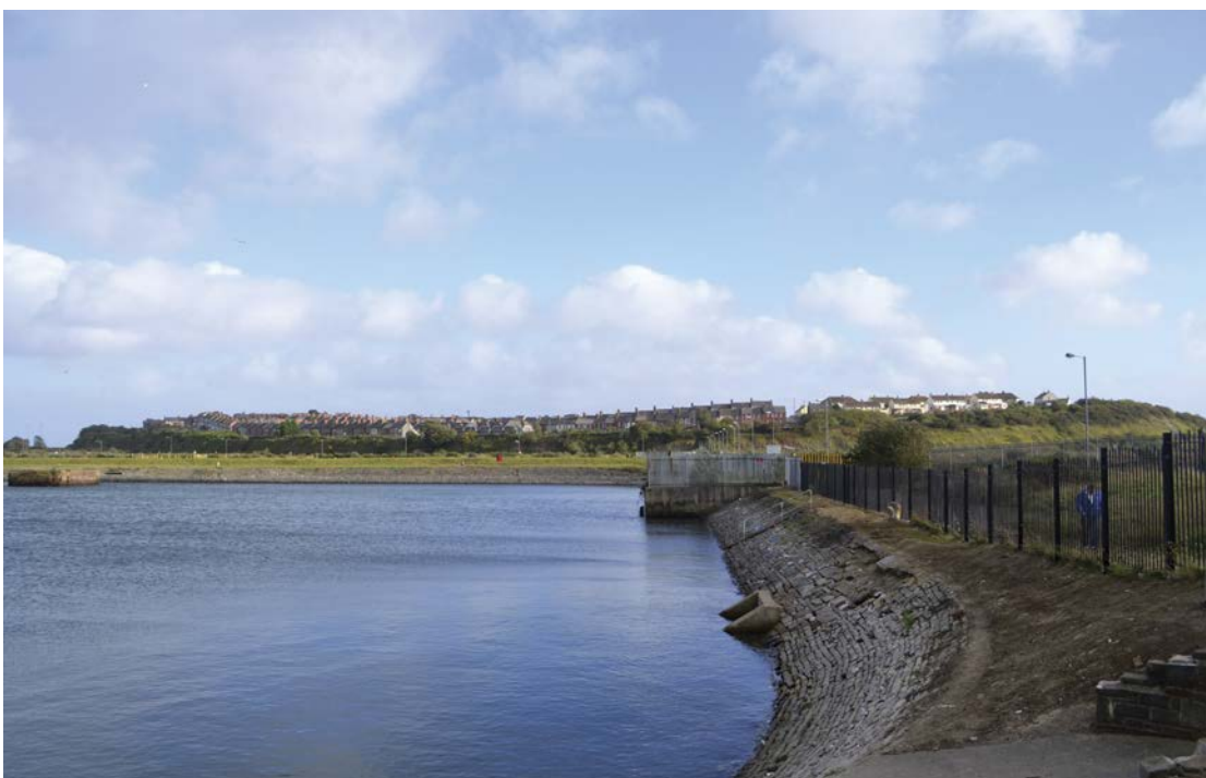
Looking from the north side of the dock towards the island's cliffs, created when the hillside was cut back to make room for the southern quay of the new docks. Photographed in September 2011 (© Civic Trust Cymru).
