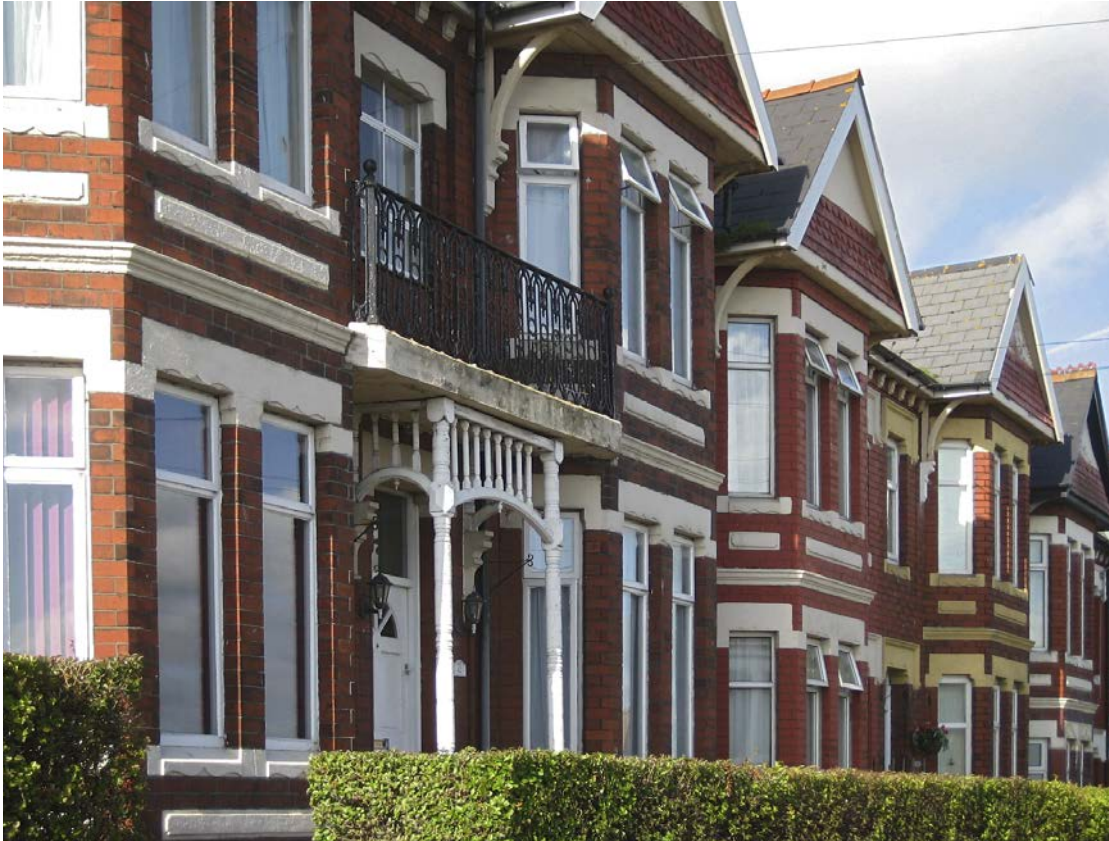
32 to 42 Redbrink Crescent have double-height bays with heavy stone detailing. Photographed in September 2011 (© Civic Trust Cymru).
