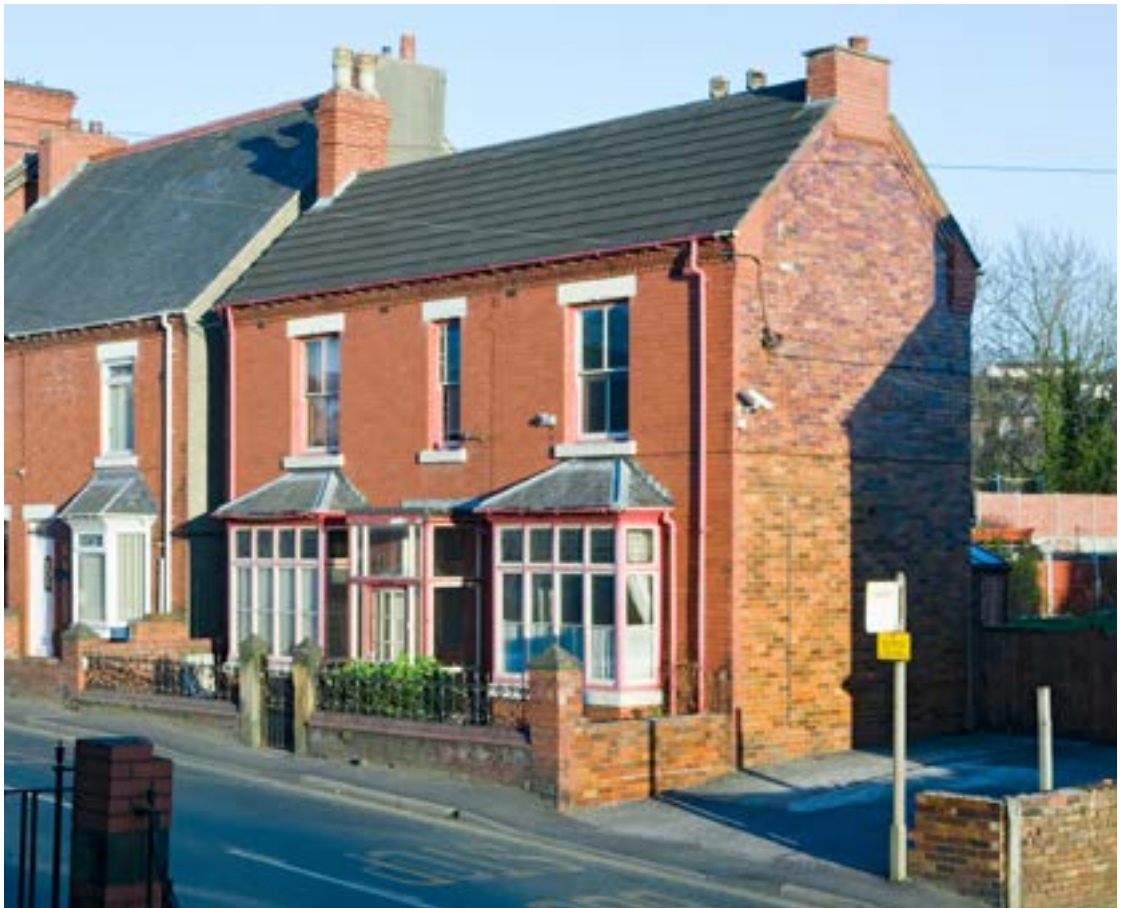
Glazed brick in the end wall of the last house in a short row on Llangollen Road (Crown Copyright: RCAHMW).
