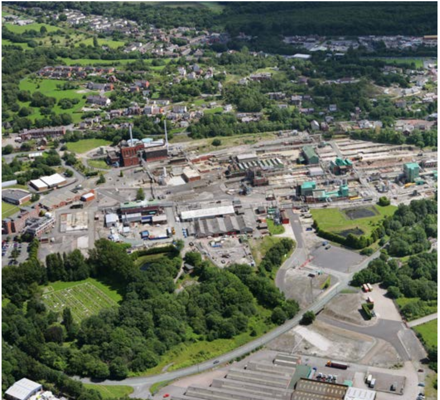
Below: The cleared site of the chemical works in 2009 (Crown Copyright: RCAHMW).
