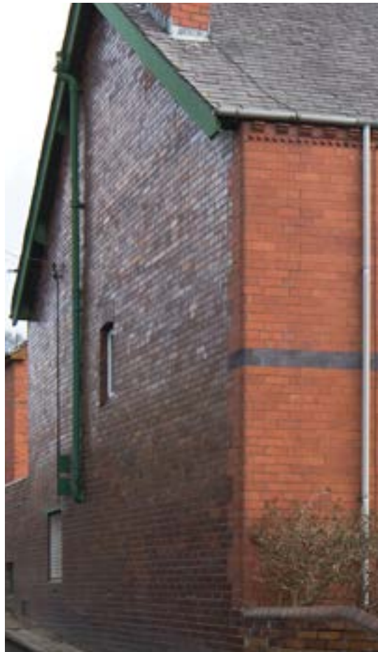
This house on Chapel Street, Acrefair, has a nicely detailed brick façade; one gable wall is stone, but the other is built of a highly-glazed brick, also used in the boundary wall (Crown Copyright: RCAHMW).
