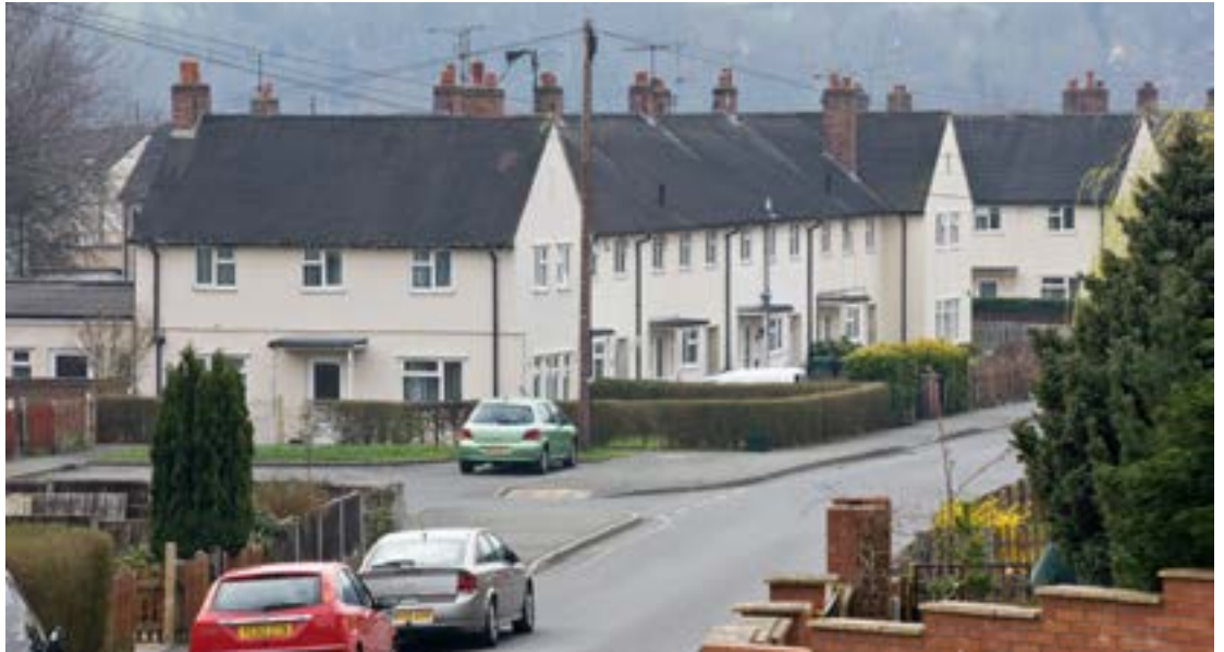
Right and below: Picturesque groupings of housing at Dolydd (Crown Copyright: RCAHMW).
