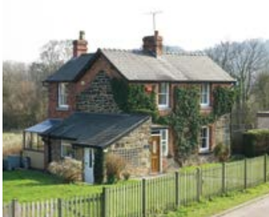
Brick used to add height to a stone cottage at Trevor basin (Crown Copyright: RCAHMW).
