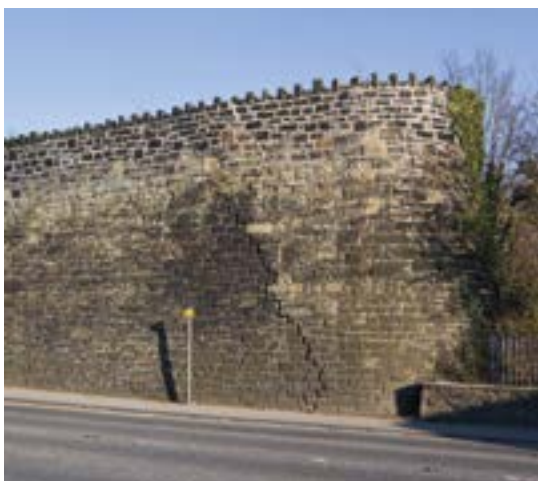
This impressive retaining wall is an important legacy of the British Ironworks (Crown Copyright: RCAHMW).
