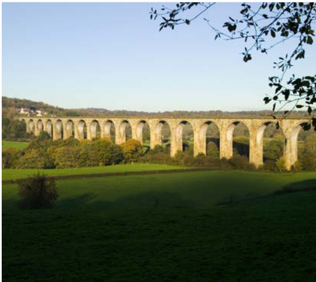
The viaduct at Newbridge in 2007 (Crown Copyright: RCAHMW).
