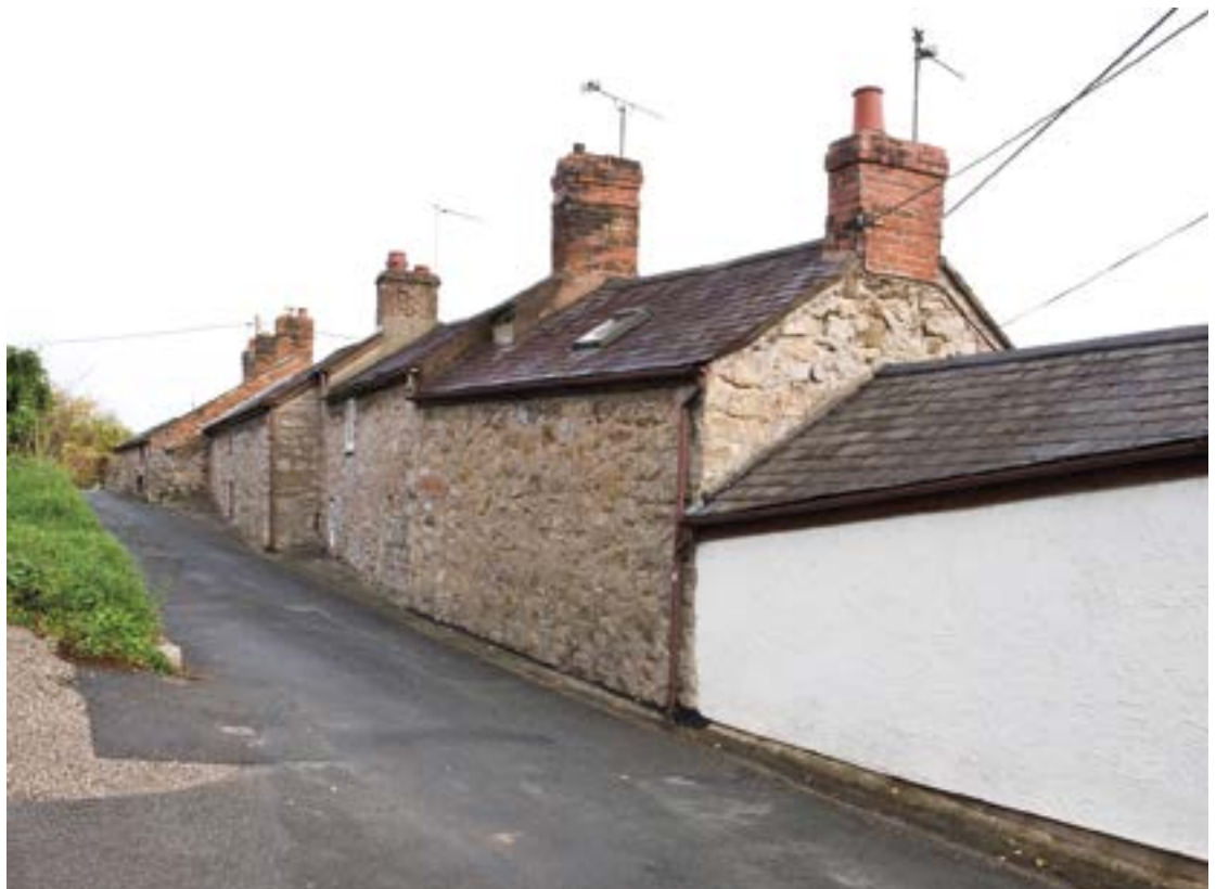
Cottages in Froncysyllte, built with their back walls right on the edge of a lane (Crown Copyright: RCAHMW).
