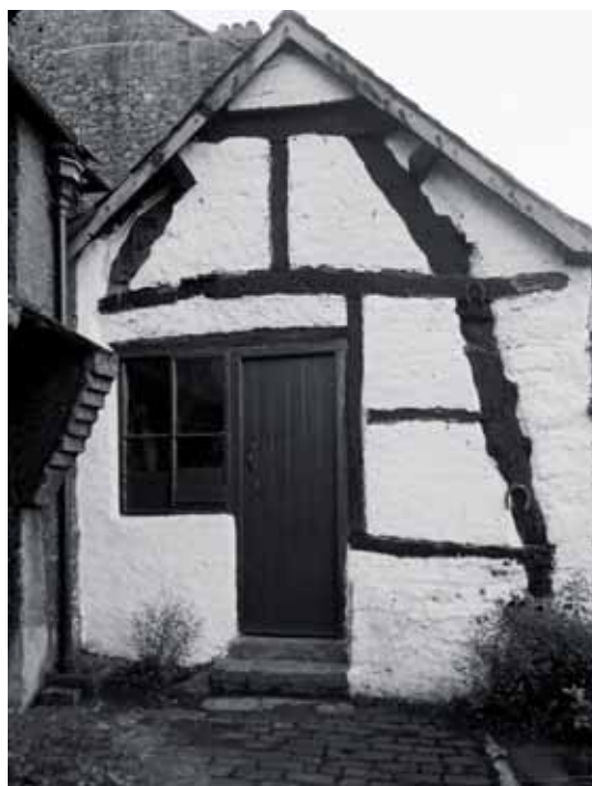
A cruck frame recorded at the back of The Old Castle Arms (Crown Copyright: RCAHMW, 1954).
