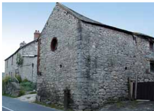
A farm building betrays the urban-edge context of Henllan Street.
