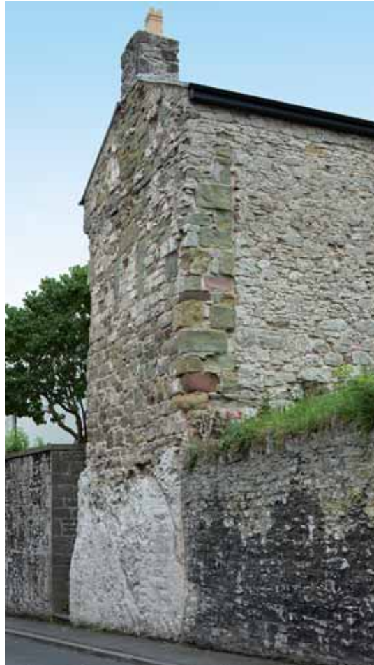
This house on Highgate may be the earliest domestic structure in the town (Crown Copyright: RCAHMW).
