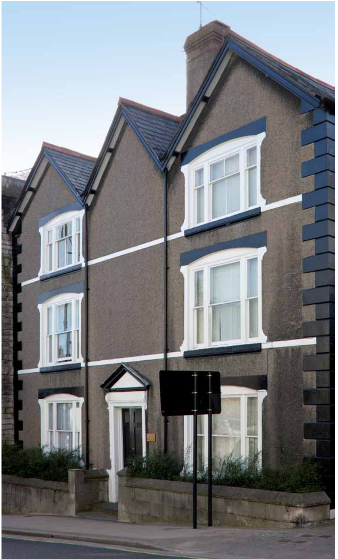
24 Vale Street is a late seventeenth-century town house with an unusual double-depth plan (Crown Copyright: RCAHMW).
