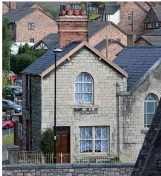
Far left: Stone and coarse render give variety to buildings on Chapel Street (Crown Copyright: RCAHMW).
