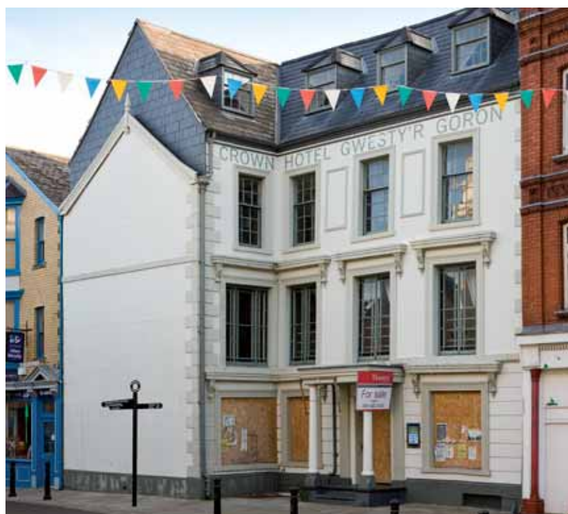
Fine render detail on The Crown Hotel (above left) and (above right) 24 High Street (Crown Copyright: RCAHMW).
