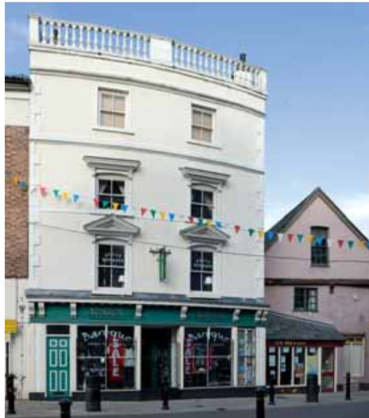
The curving façade of 13 Crown Square: a sophisticated commercial building of the nineteenth century (Crown Copyright: RCAHMW).
