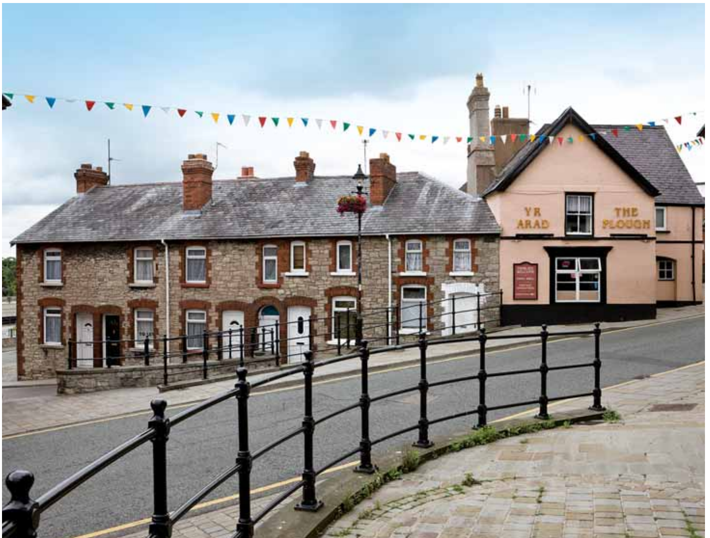
Below: Limestone rubble with brick dressings off Portland Place (Crown Copyright: RCAHMW).
