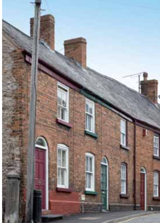
Limestone rubble walls and a brick façade on Chapel Street (Crown Copyright: RCAHMW).
