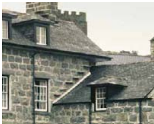
Far left: A rare surviving example of graded slate, Meyrick Street.
