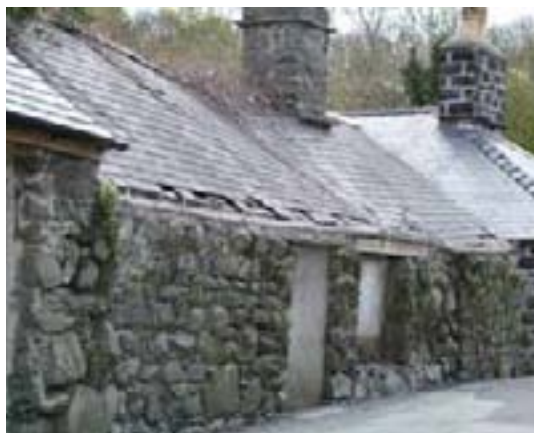
Above: Limewash on an ancillary building at Coed Wenallt.
