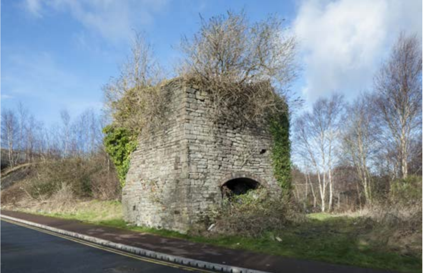
Above: The limekiln at Hafod, where lime used as the flux in the initial roasting of copper ore was prepared (© Crown Copyright: RCAHMW).
