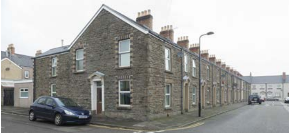
Right: A corner house on Graham Street, unusual for having the entrance in the gable end` (© Crown Copyright: RCAHMW).
