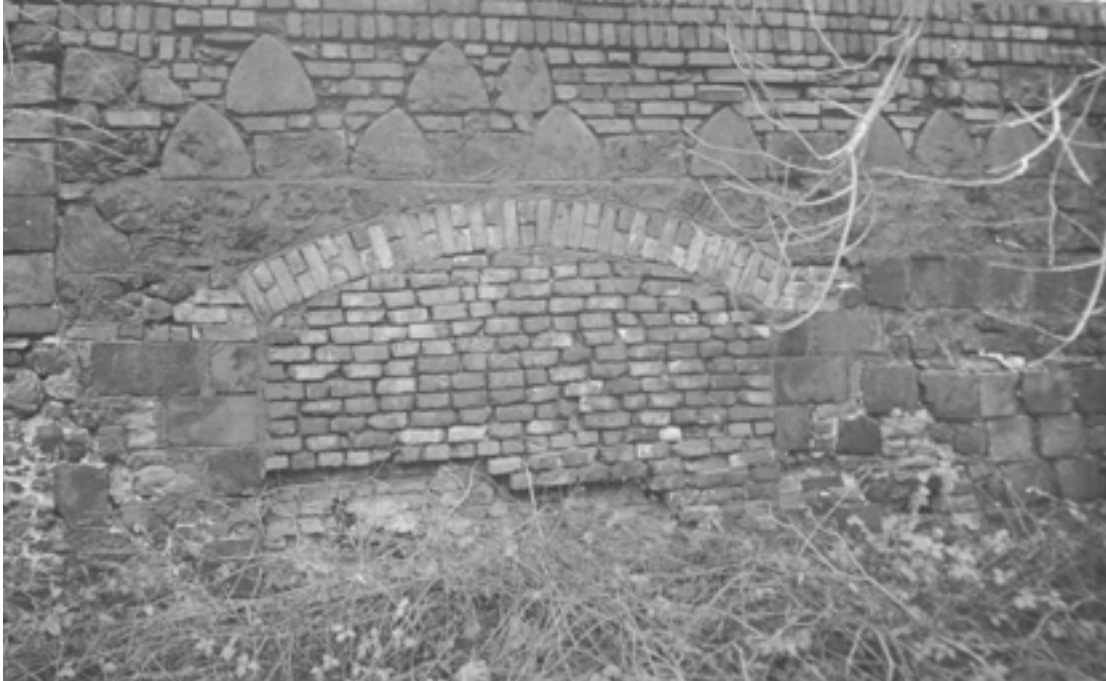
Left: Slag blocks in the entrance to the canal dock in the boundary wall of the Hafod works (© Crown Copyright: RCAHMW).
