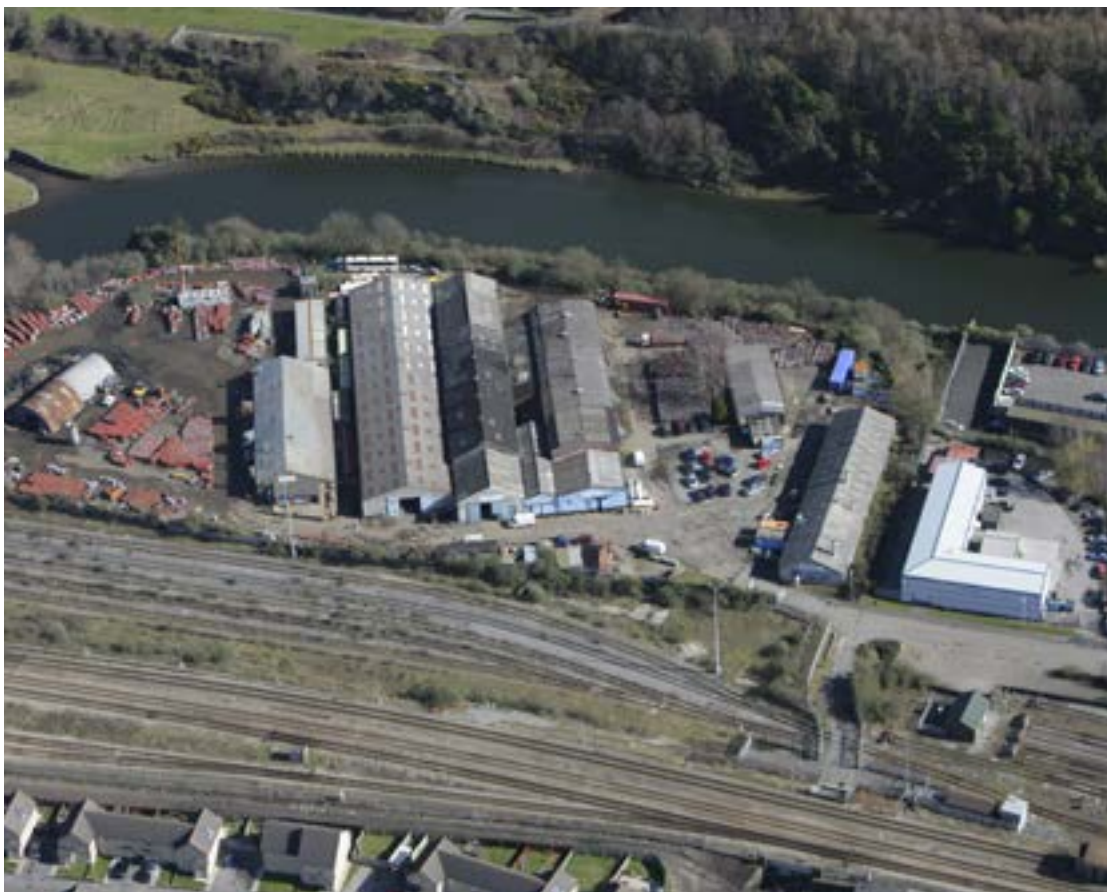
Left: This area was once busy with industries developed alongside the canal (© Crown Copyright: RCAHMW).
