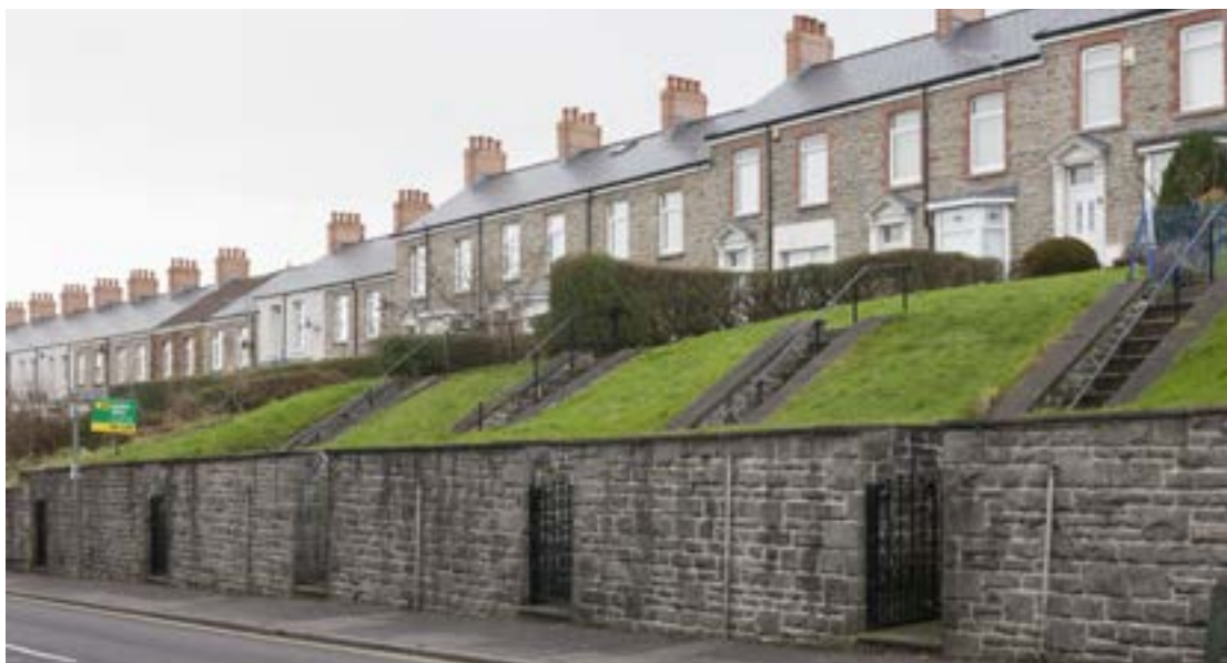
Left: Retaining walls and steep steps to front gardens, also on Neath Road (© Crown Copyright: RCAHMW).
