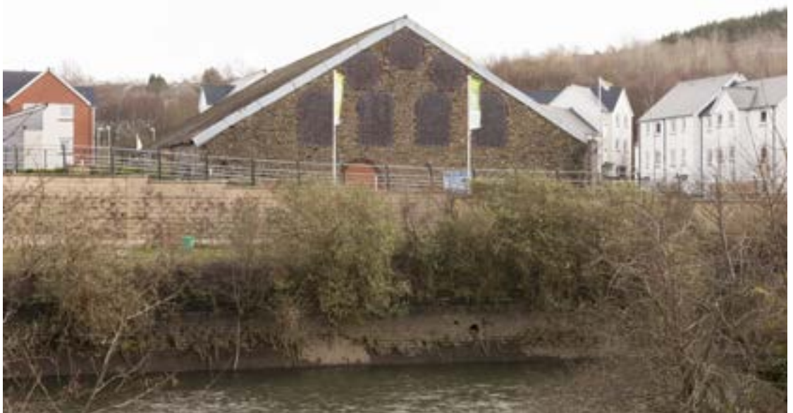
The smelting hall at Upper Bank is the only surviving example of this important industrial building type in the area (© Crown Copyright: RCAHMW).
