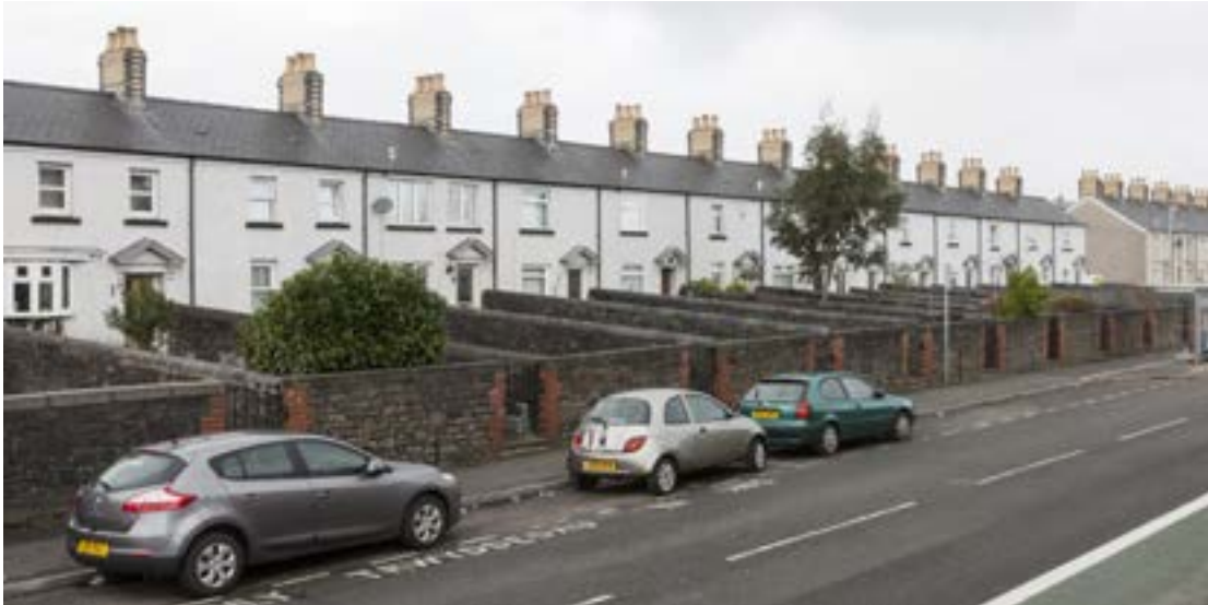
Left: Long front gardens with their distinctive boundary walls on Neath Road; (© Crown Copyright: RCAHMW).
