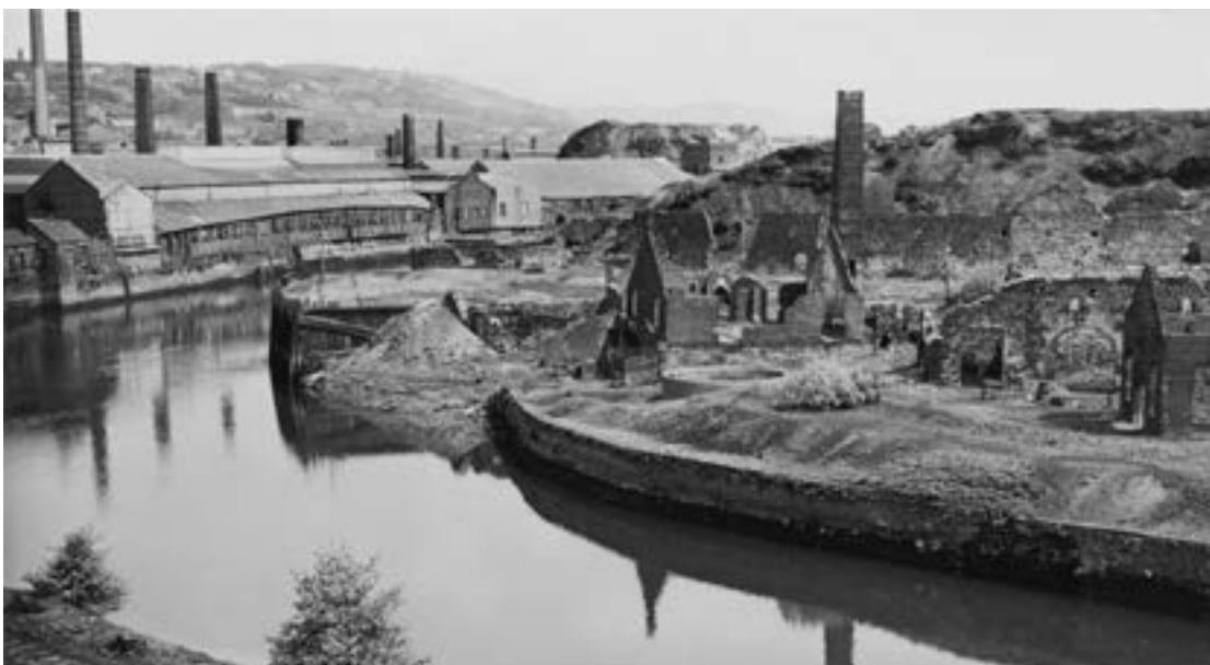
The Hafod works and the ruins of the White Rock works in the 1960s (© Crown Copyright: RCAHMW).
