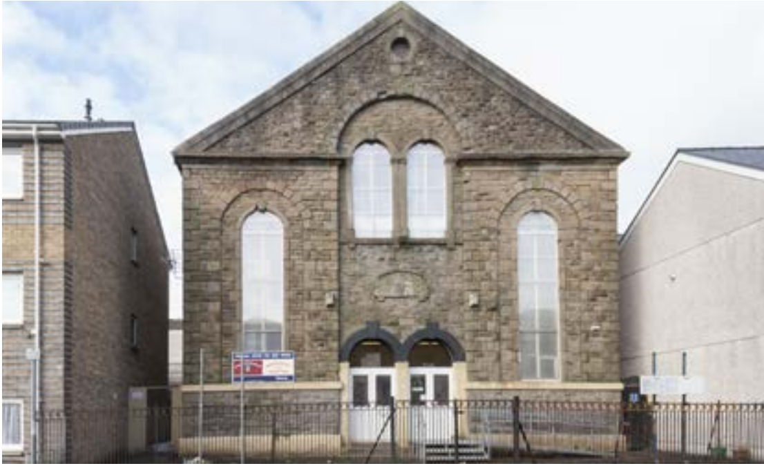
Philadelphia Chapel was built in 1867 (© Crown Copyright: RCAHMW).
