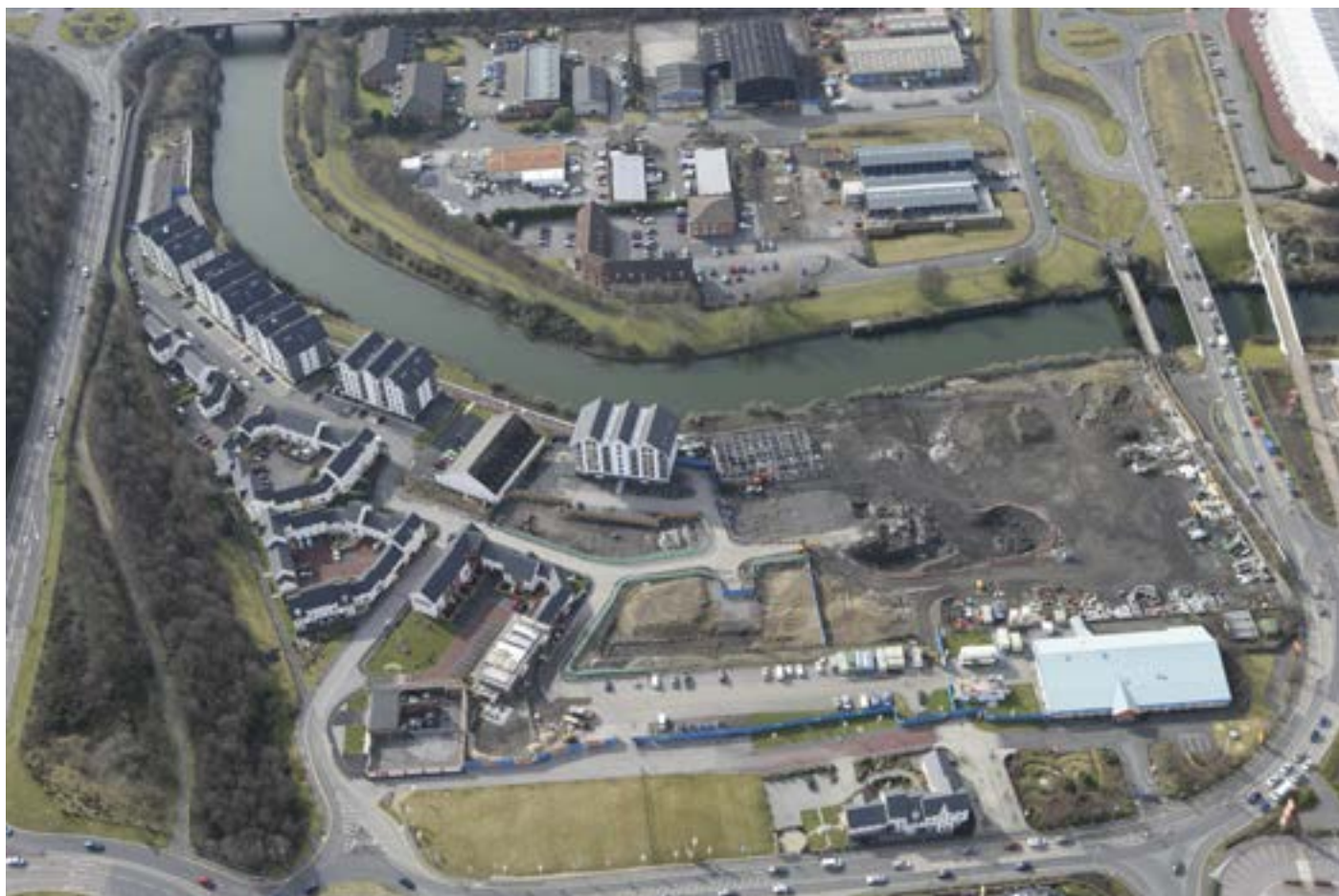
The site of the Upper Bank Copperworks in 2010 (© Crown Copyright: RCAHMMW).
