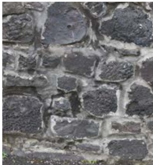
Left and middle: Copper slag as a walling material, or cast into blocks for copings, is a distinctive local material (© Crown Copyright: RCAHMW).
