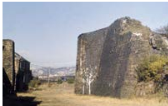
Left and below: These abutments once supported an inclined plane (© Crown Copyright: RCAHMW).
