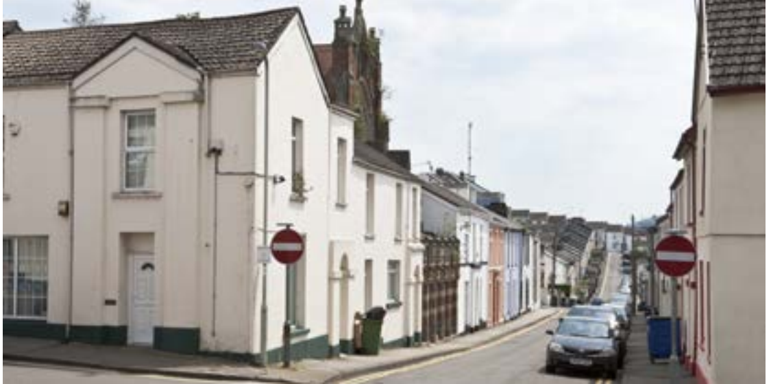
Formal treatment to the corner building on Upper Thomas Street (Crown Copyright: RCAHMW).
