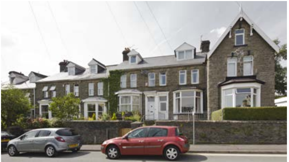
Larger terraced houses with small front gardens on Park Terrace (right) and Norman Terrace (below) (Crown Copyright: RCAHMW).
