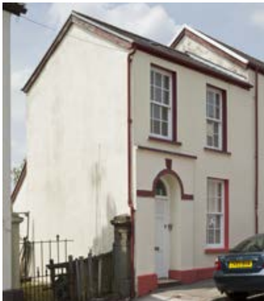
Smooth rendered finish and simple classical detail on houses on Lower and Upper Thomas Street (Crown Copyright: RCAHMW).
