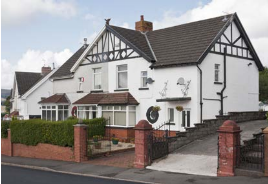
The northern part of this area favoured large suburban housing like these examples at Pembroke Place (Crown Copyright: RCAHMW).
