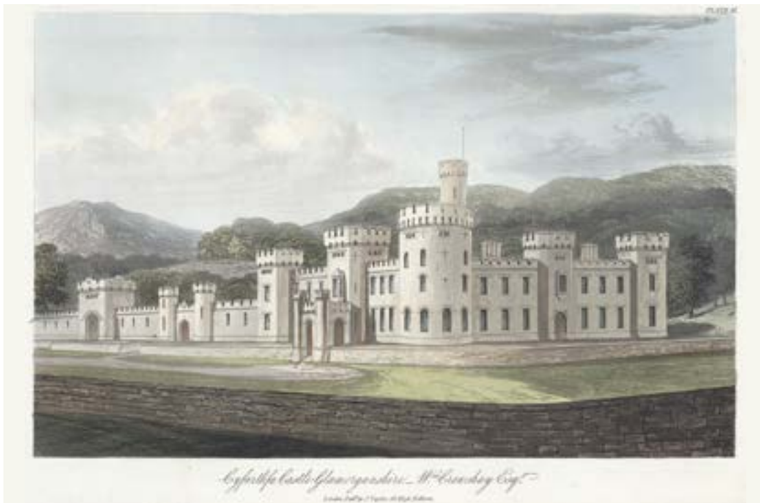
Pennant Sandstone was the main building material used at Cyfarthfa Castle (above), but Carboniferous Limestone was also used here. The castle is shown gleaming white in this picture of about 1840 (By permission of Llyfrgell Genedlaethol National Library of Wales; Crown Copyright: RCAHMW).
