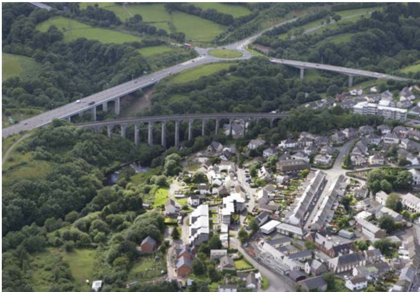
The viaduct at Cefn Coed, with the Heads of the Valleys road and A470 in the background. (Crown Copyright: RCAHMW).
