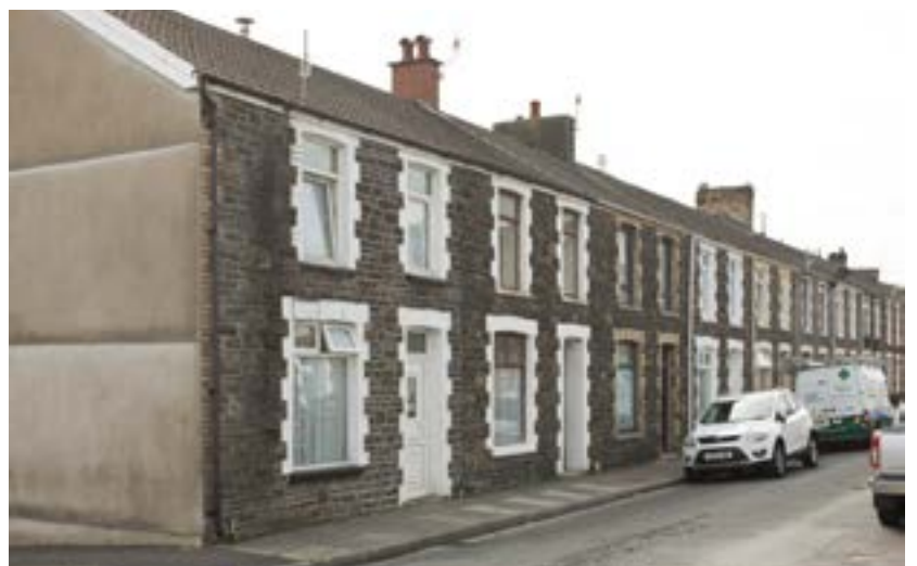
Below: Planned development: Stuart Street (Crown Copyright: RCAHMW).
