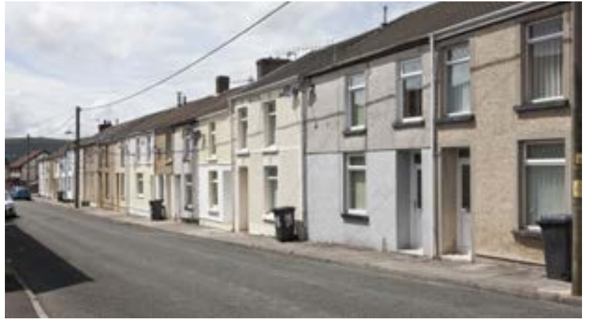
Some of the housing associated with Penydarren Ironworks: Church Street, Penydarren (Crown Copyright: RCAHMW).
