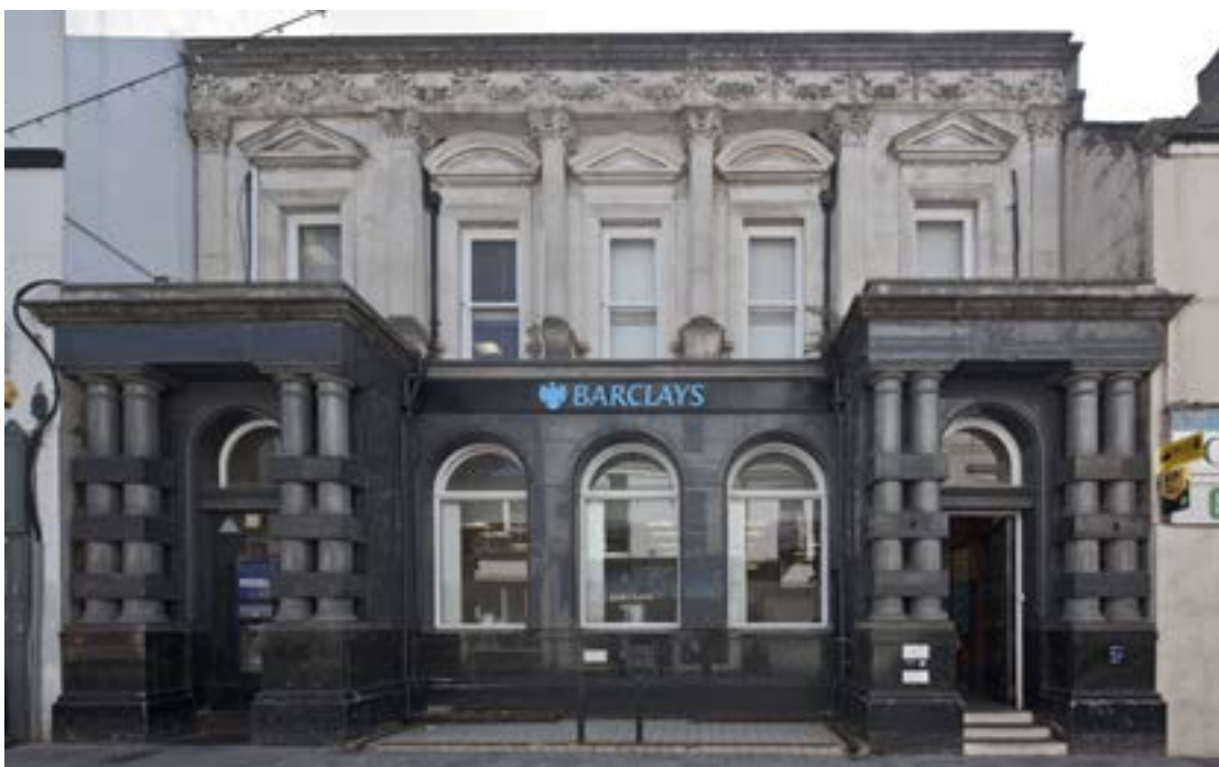
The status of this bank building is demonstrated by the use of expensive imported materials (Crown Copyright: RCAHMW).
