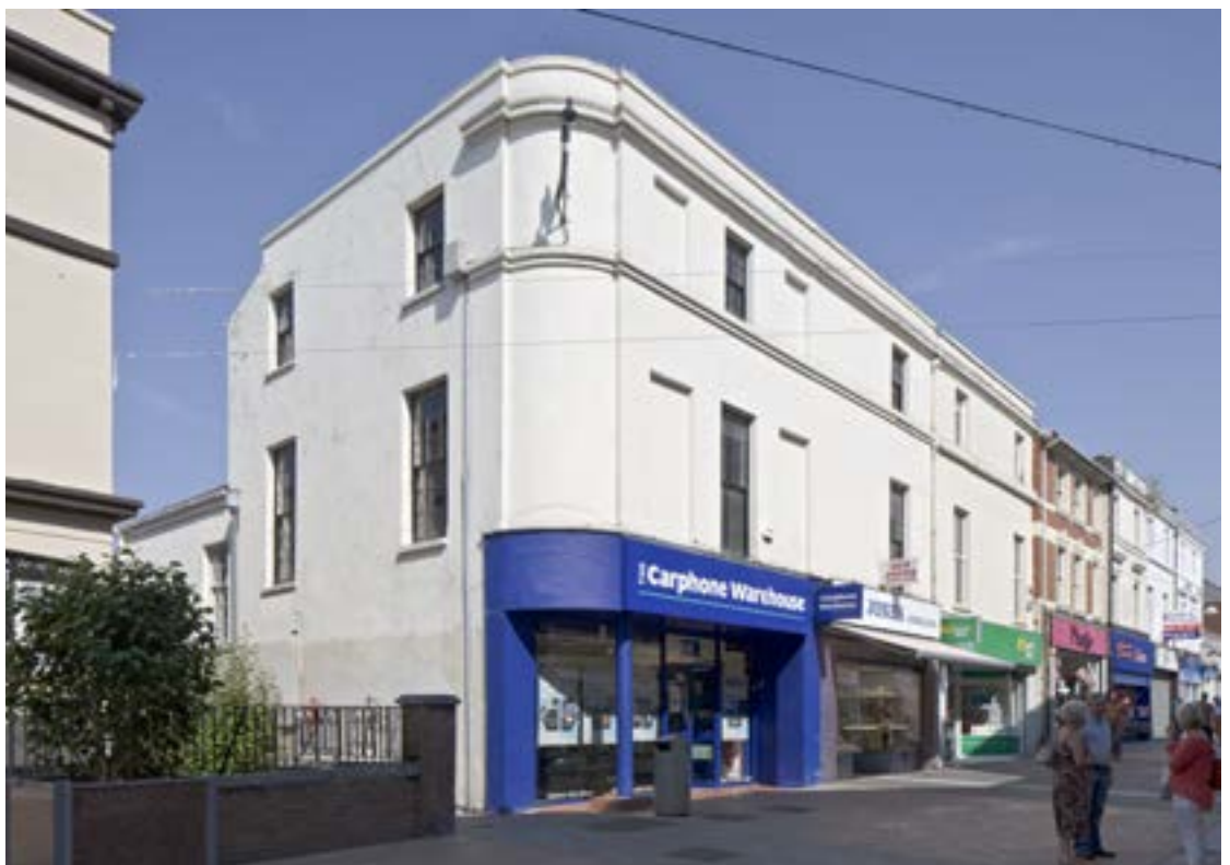
A corner has been given architectural treatment in this mid-nineteenth-century commercial building, which is also a good example of the fashion for render in that period (Crown Copyright: RCAHMW).
