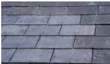
Above and left: There are some good examples of PV roof cladding that emulate the look of natural slate and the technology is constantly evolving. The slates pictured have the advantage of being thin and non-reflective, though rarely will they be a suitable substitute for Welsh slate on a principal roof slope.
