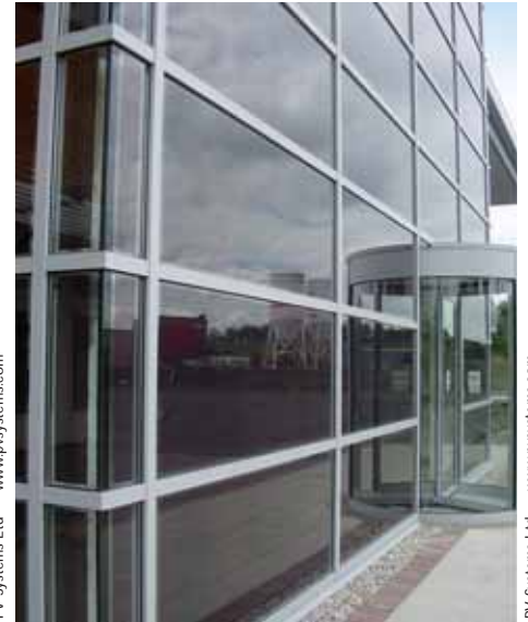
Above left and right: Amorphous silicon cells can be used to coat glass. This example is on a new building, but this type of glass set into a well-designed frame could be used to good effect on historic buildings where large areas of new glazing are proposed, such as a threshing barn that is being converted to domestic use.
