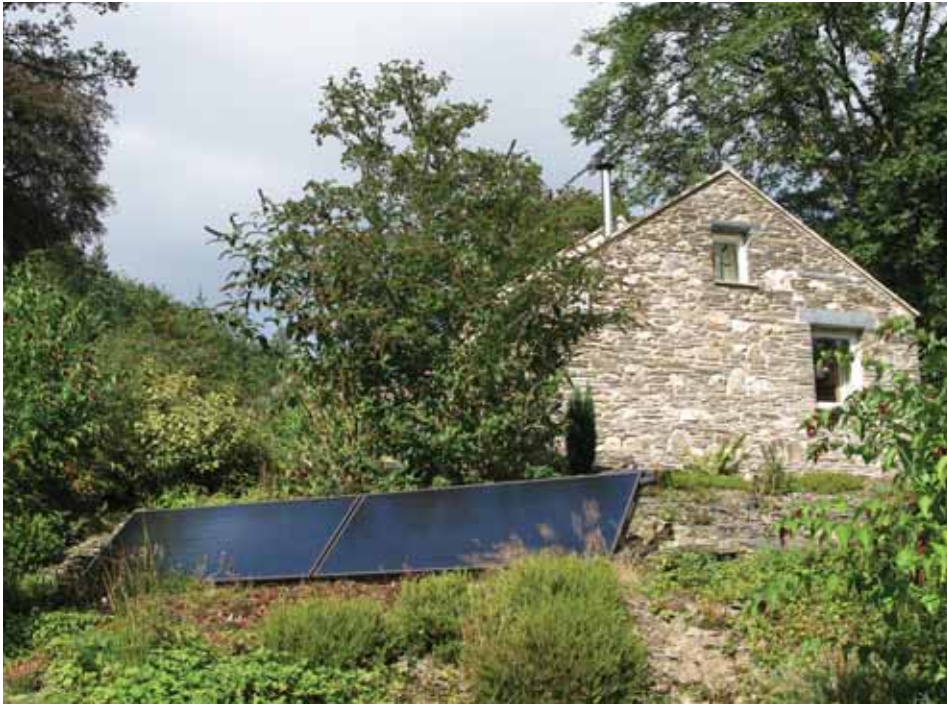
These free-standing solar hot-water panels have been carefully sited so as to blend in with the surrounding rockery and planting scheme.
