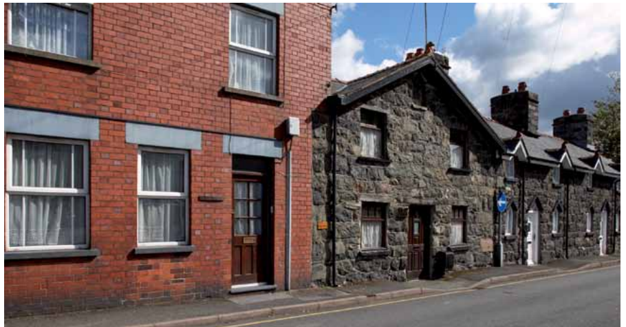
3 Houses in Mount Street show the transition from local stone to brick after the railway came to Bala in 1868
