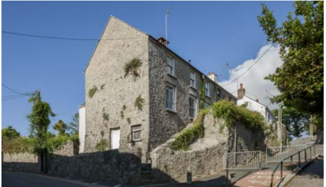
Prospect House and cottage (1 and 2 Church Terrace): a probable seventeenth-century pair of buildings with a large external chimney stack surviving to the right gable. Both buildings have been later altered (Crown Copyright: RCAHMW).
