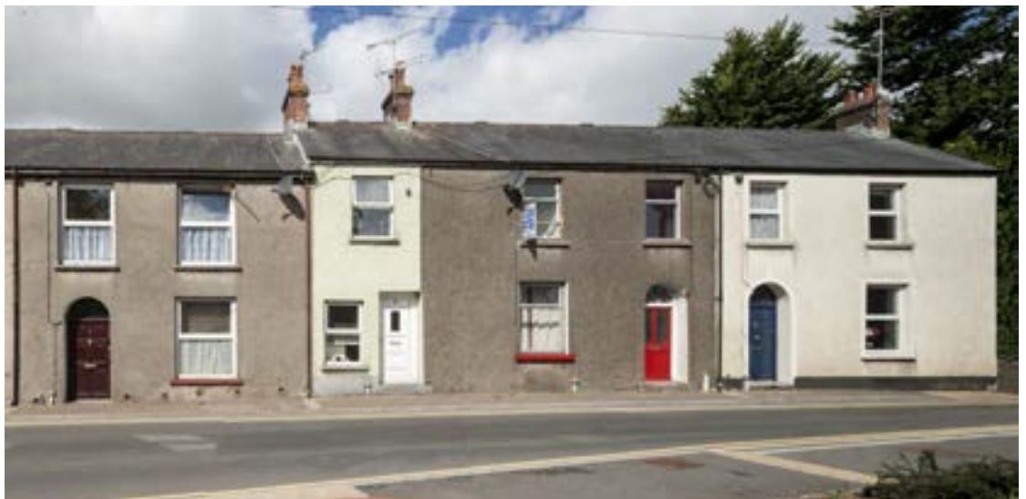
School Terrace, from the southern end of Bridgend Terrace. 2 retains an original fanlight. 3, to the left, demonstrates an efficient use of space between two other houses (Crown Copyright: RCAHMW).
