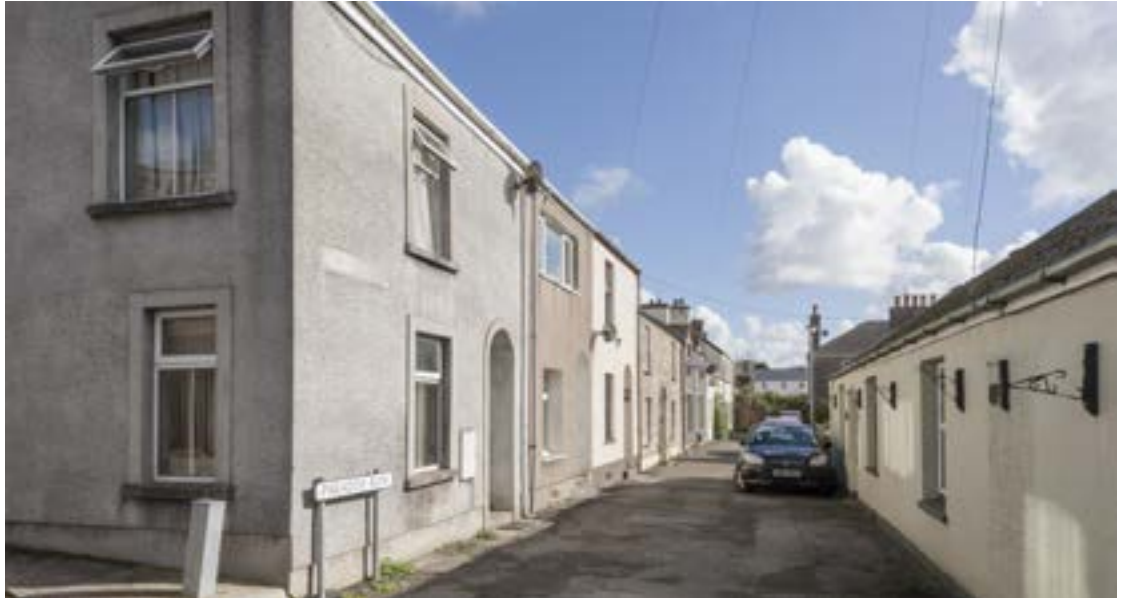
Paradise Row (Crown Copyright: RCAHMW).
