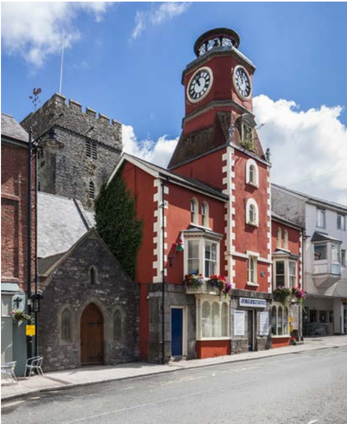
The Clock Tower or Clock House. Originally constructed in the early nineteenth century, the low wings to either side have been heightened and altered twice; the tower itself was altered in 1899 (Crown Copyright: RCAHMW).
