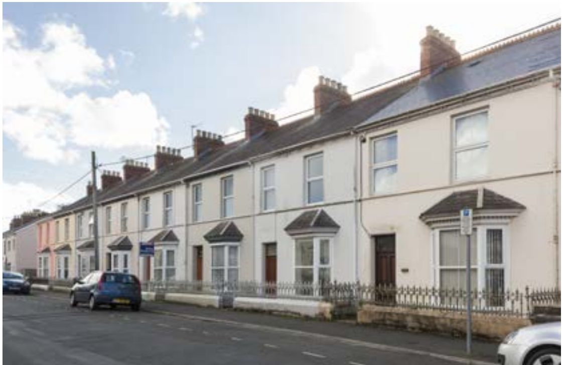
1–8 Woodbine Terrace (Crown Copyright: RCAHMW).
