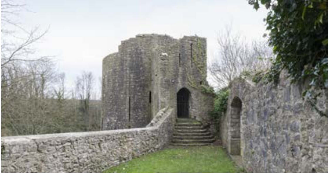
Barnard's Tower on the north-eastern circuit of the walls (Crown Copyright: RCAHMW).
