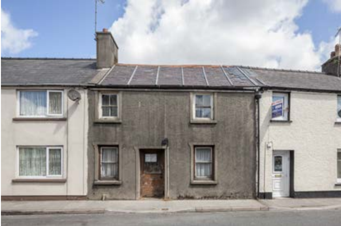
A rendered house with a cement-based roughcast and raised window architraves formed in render (Crown Copyright: RCAHMW).
