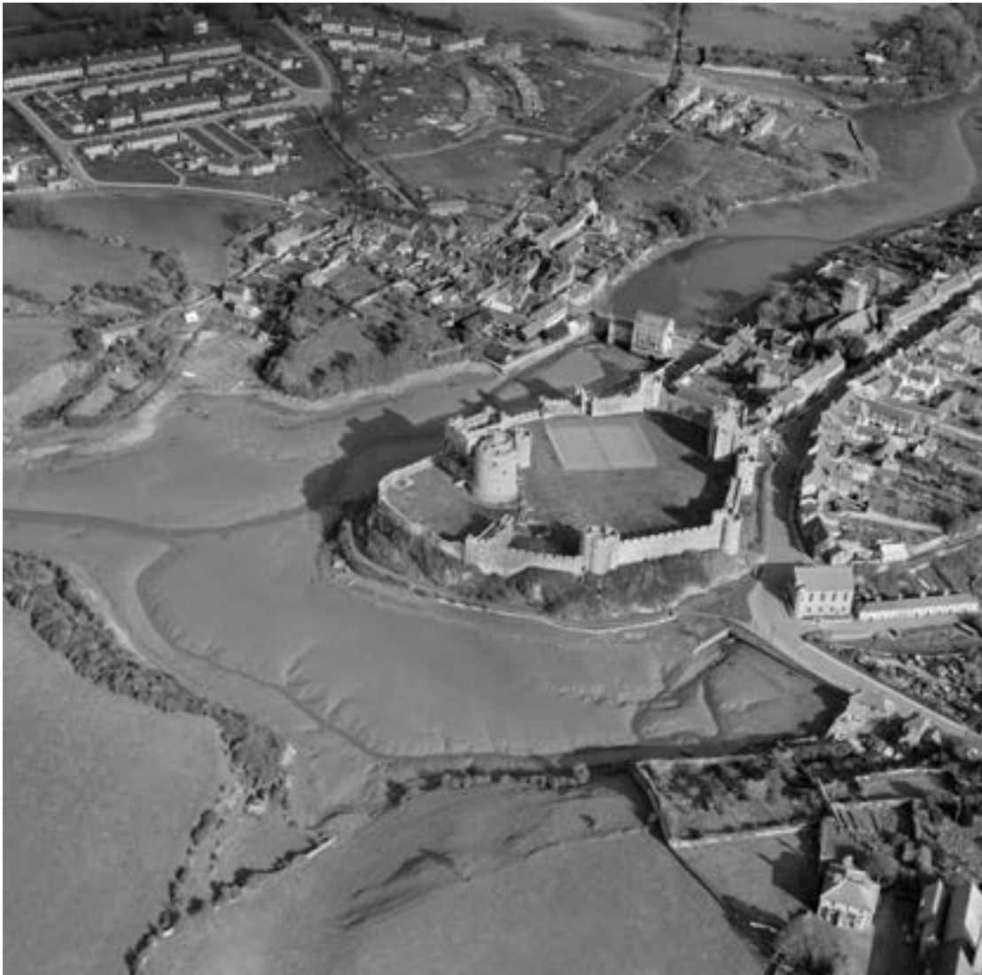
A 1950 view of the castle and the town with the suburb of the Green across Mill Bridge and the newly laid-out estate of housing to the north and east (Crown Copyright: RCAHMW).
