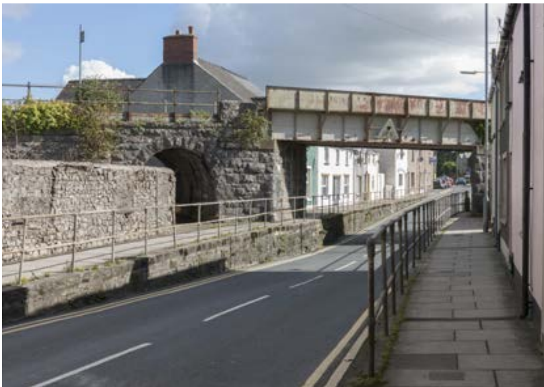
The elevated railway line crossing over Station Road (Crown Copyright: RCAHMW).
