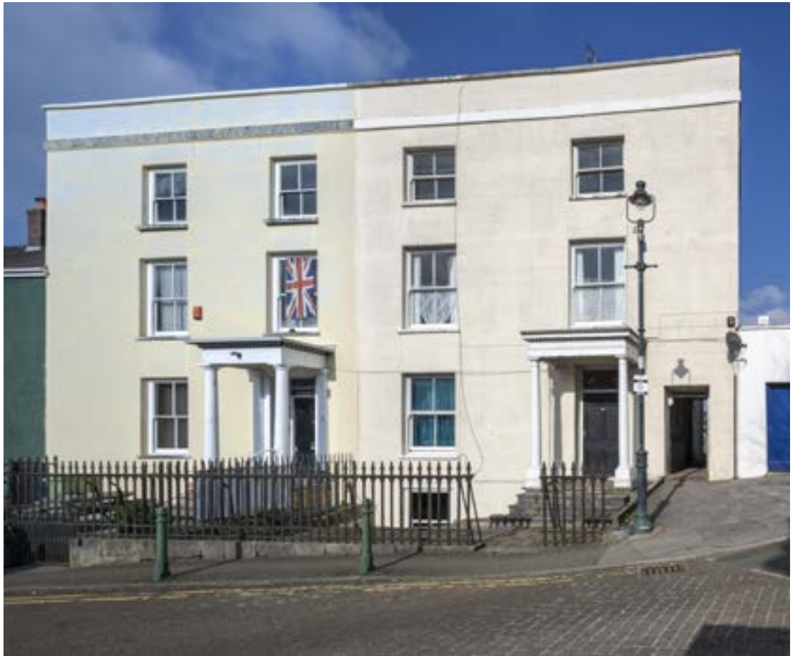
Late Georgian housing. 86 and 88 Main Street is a pair of semi-detached early nineteenth-century houses, probably built by the Orielton estate (Crown Copyright: RCAHMW).
