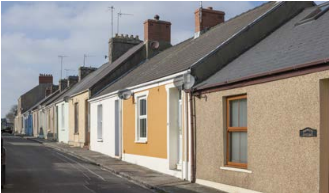
Orange Gardens housing: 5–14 Owen Street (Crown Copyright: RCAHMW).
