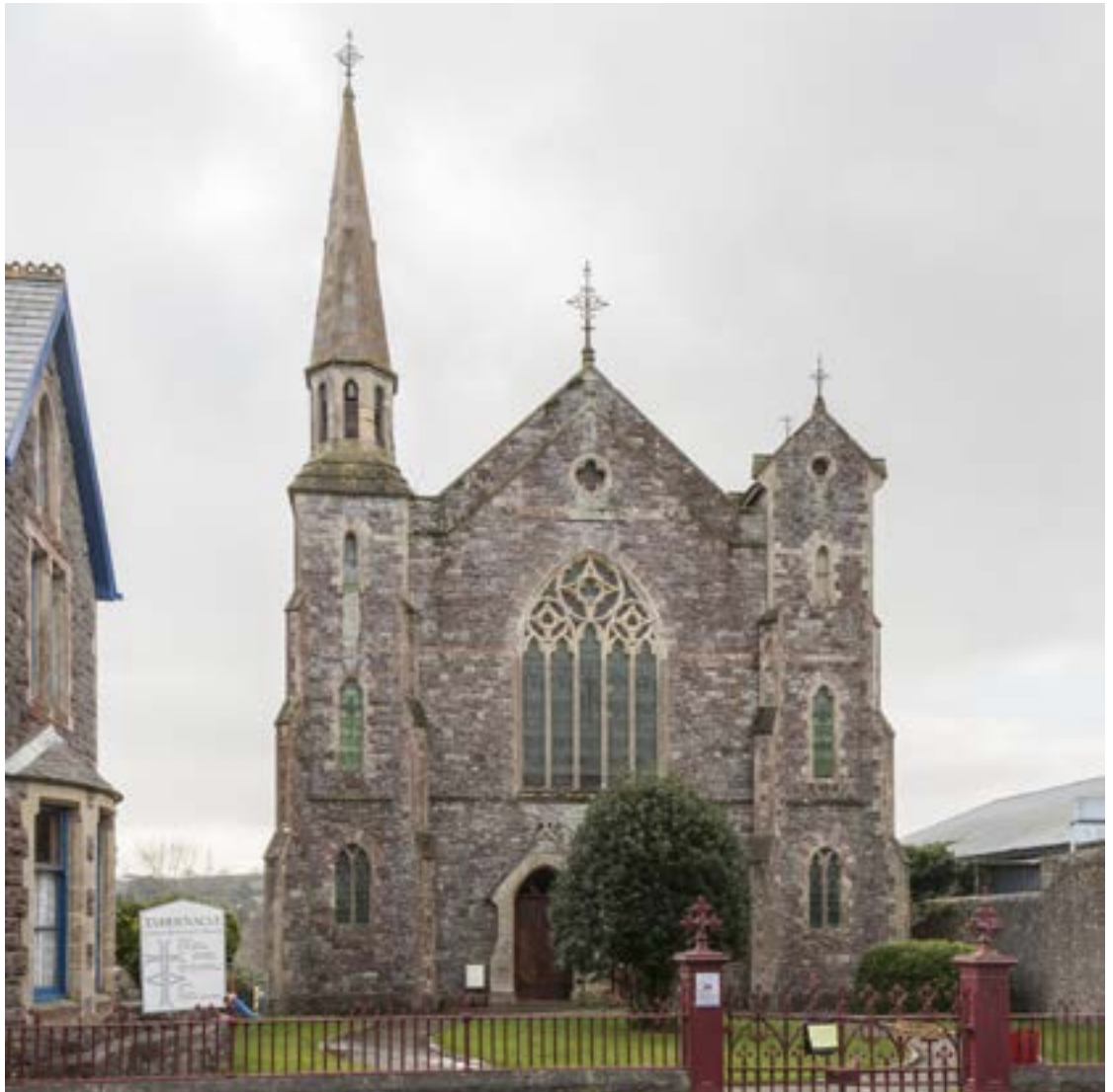
The Tabernacle United Reformed (formerly Congregational) Church on Main Street (Crown Copyright: RCAHMW).
