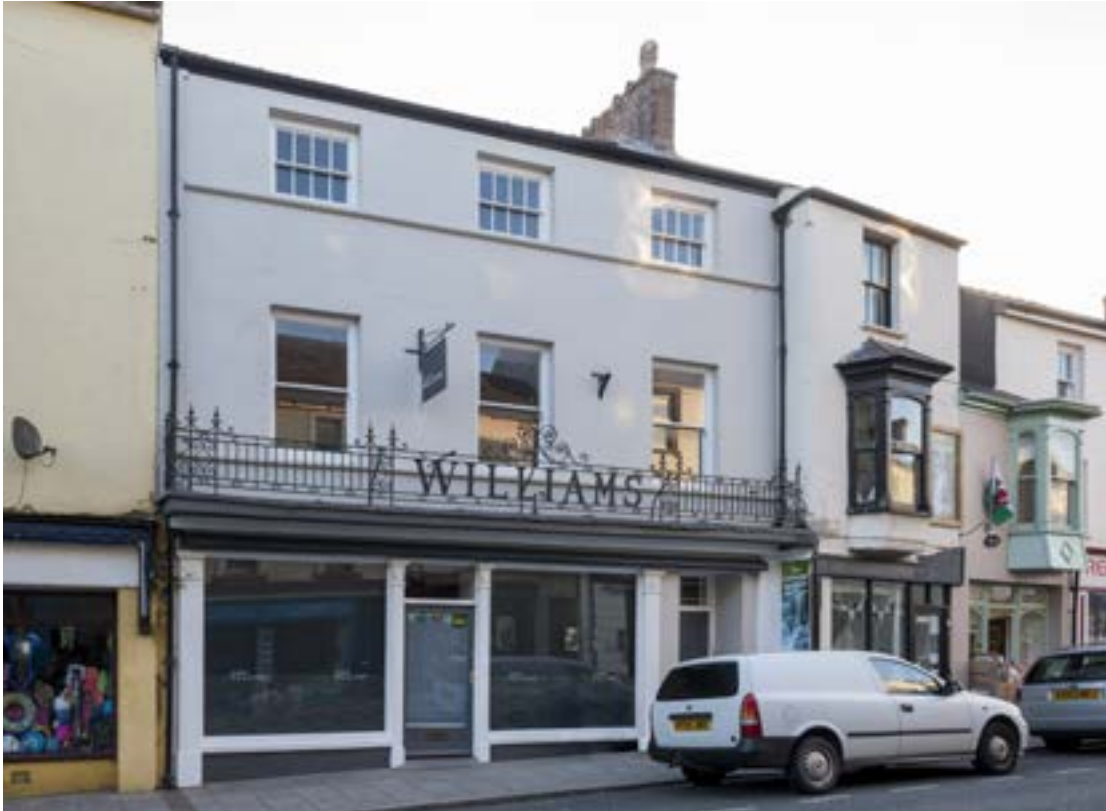
18 Main Street. An early nineteenth-century terraced house, which was altered in the late nineteenth century when the ground floor became a shop. At the same time, large pane sash windows were inserted on the first floor together with decorative ironwork which survives above the shopfront. There was also a broad canopy over the pavement but this has not survived (Crown Copyright: RCAHMW).
