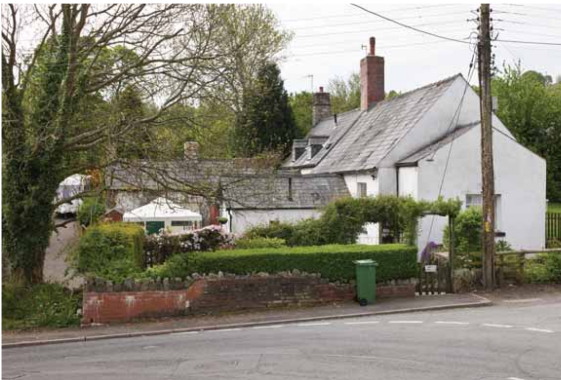
An older survival on Twmpath Road (Crown Copyright: RCAHMW).
