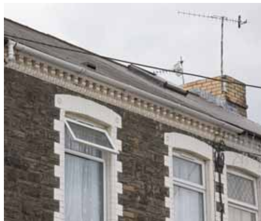
Rock-faced rubble combined with brick and terracotta (Crown Copyright: RCAHMW).
