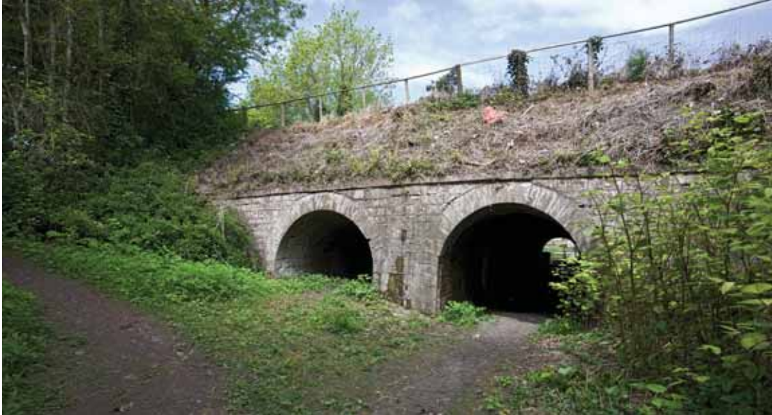
These arches once took a tram road and a water supply underneath the canal to the tinplate works at Lower Mill (Crown Copyright: RCAHMW).
