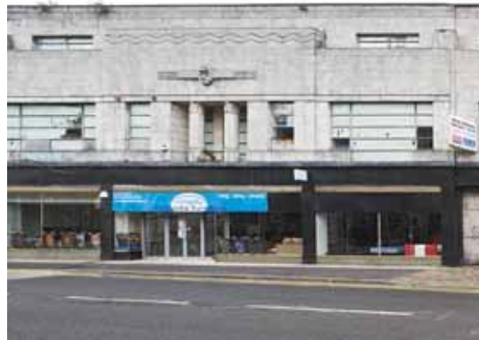
Far left: The former Clarence Hotel (Crown Copyright: RCAHMW).
