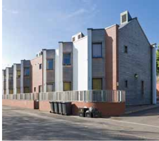
Far left: Modest terraced houses characterize the northern end of Osborne Road (Crown Copyright: RCAHMW).
