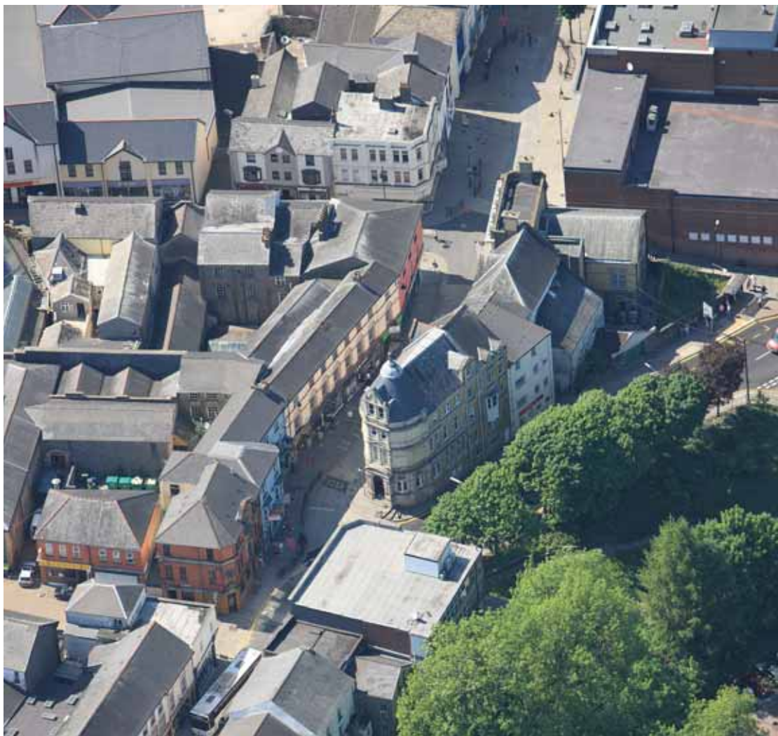
Dense development patterns in the town centre (Crown Copyright: RCAHMW).
