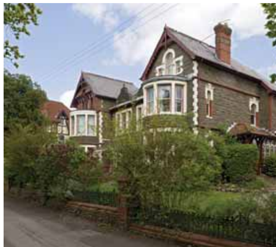
Inter-war public housing at Penygarn (Crown Copyright: RCAHMW).
