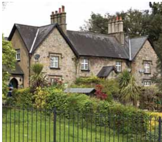
Far left: An early vernacular building at Maesderwen (Crown Copyright: RCAHMW).
