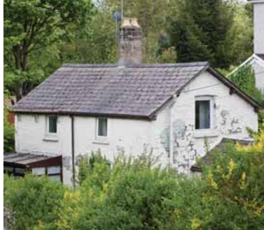
Far left: An eighteenth-century house, thought to have been used as the truck house of the Monmouthshire Canal Company in the nineteenth century, with early nineteenth-century terraced houses beyond (Crown Copyright: RCAHMW).
