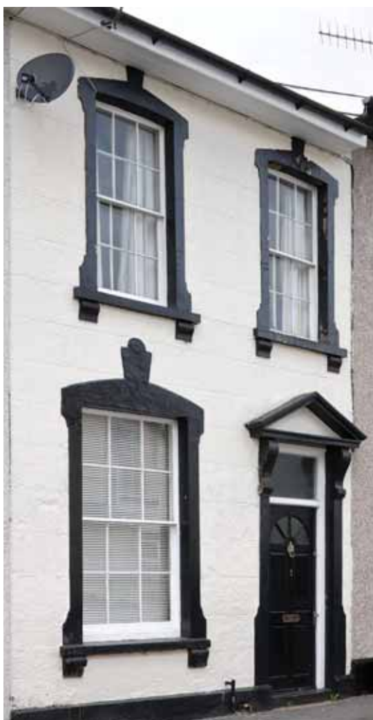
Right: A surviving example of scribed render (Crown Copyright: RCAHMMW).
