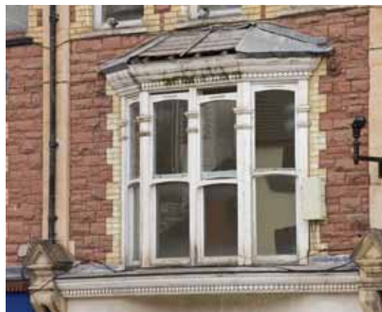
Left: Surviving original detail on Osborne Road (Crown Copyright: RCAHMW).
