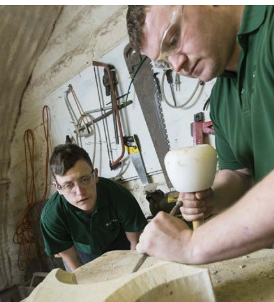
Cadw stonemasons carving replacement stone tracery.
