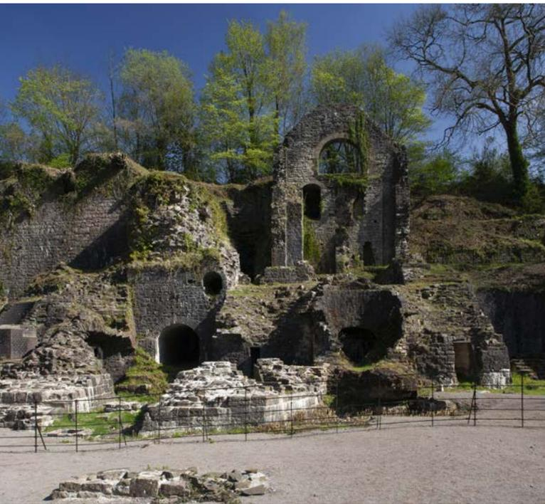
Clydach Ironworks, Monmouthshire. Founded between 1793 and 1795, the ironworks had four blast furnaces, associated charging-houses and a cast house. A counter-balanced railway inclined plane enabled pig iron to be lifted to the rolling mills located on higher ground to the east of the ironworks. The ironworks has the potential to enhance our knowledge and understanding of the development of the iron industry in south Wales, especially as it is part of a larger industrial landscape.
