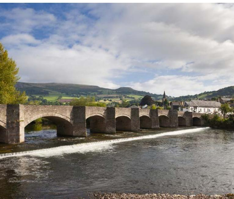
Crickhowell Bridge, Powys. This stone bridge was built in 1706 to carry the single carriageway road across the River Usk. It was widened in 1810 when two of the arches at the north-east end were merged into one, resulting in 12 arches on the northern, upstream, side and 13 arches on the southern, downstream, side. The bridge is important because it may help us to better understand post-medieval construction techniques and transportation systems.
