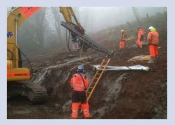
Repairs to the embankment near Llanfoist. © Canal and River Trust
