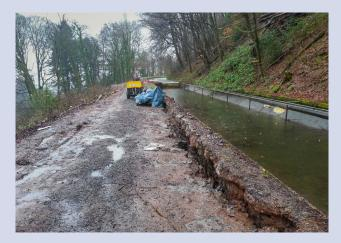
Grounding slumping away from the concrete lining of the canal near Tod's Bridge. © Canal and River Trust
