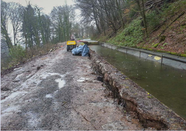
Grounding slumping away from the concrete lining of the canal near Tod's Bridge.
