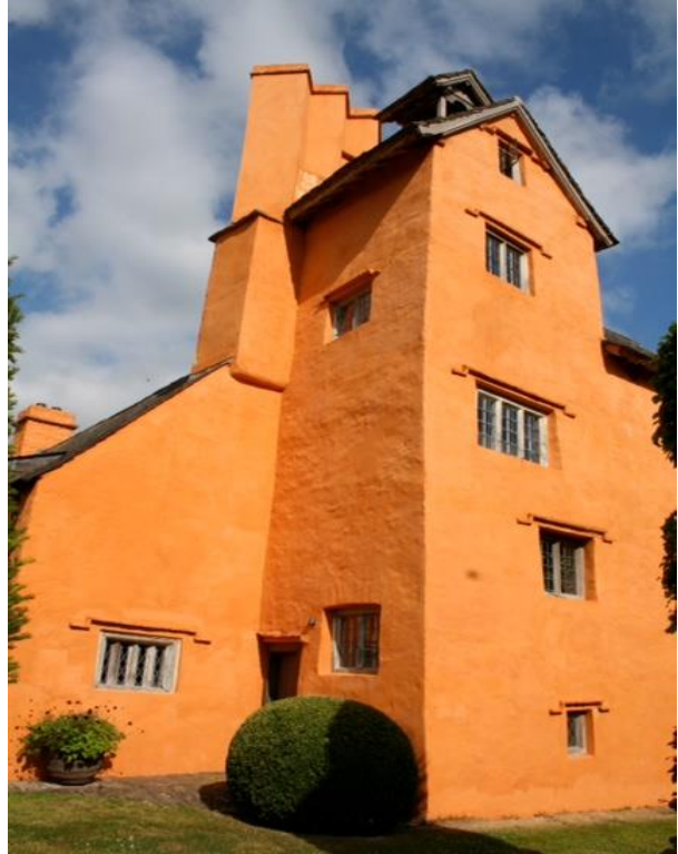
Allt y Bela c.2018 after restoration
