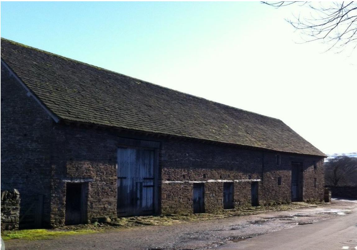
Tretower Barn before restoration project began.
