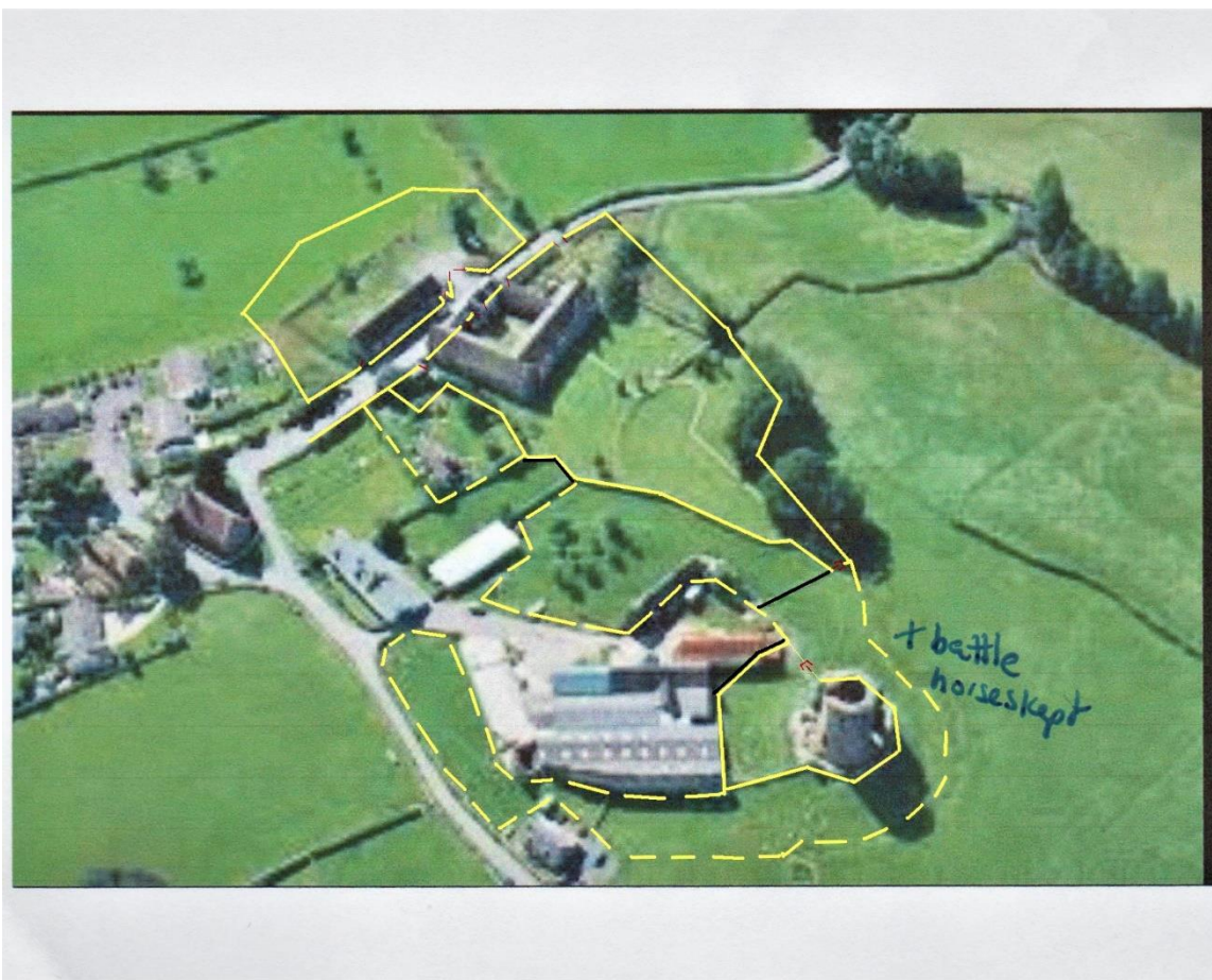
Tretower Court and Castle Aerial View.
