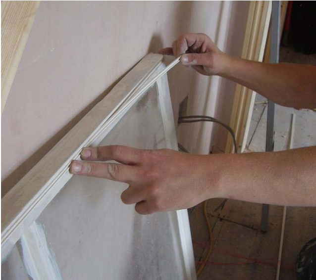
Figure 12: Draught proofing is a quick low-cost measure that will significantly improve energy efficiency (© Core Sash Windows).
