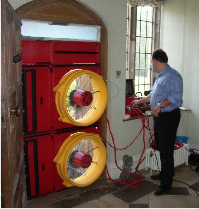
Figure 10: Air pressurisation tests are used to determine the airtightness of the building and the amount of air leaking out of the building envelope (© Oxley Conservation).
