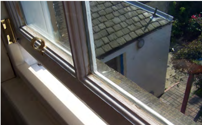
Left: The original timber window frame can accommodate new double-glazing, making the change visually discrete. Next page: Double glazed units in sash windows.
