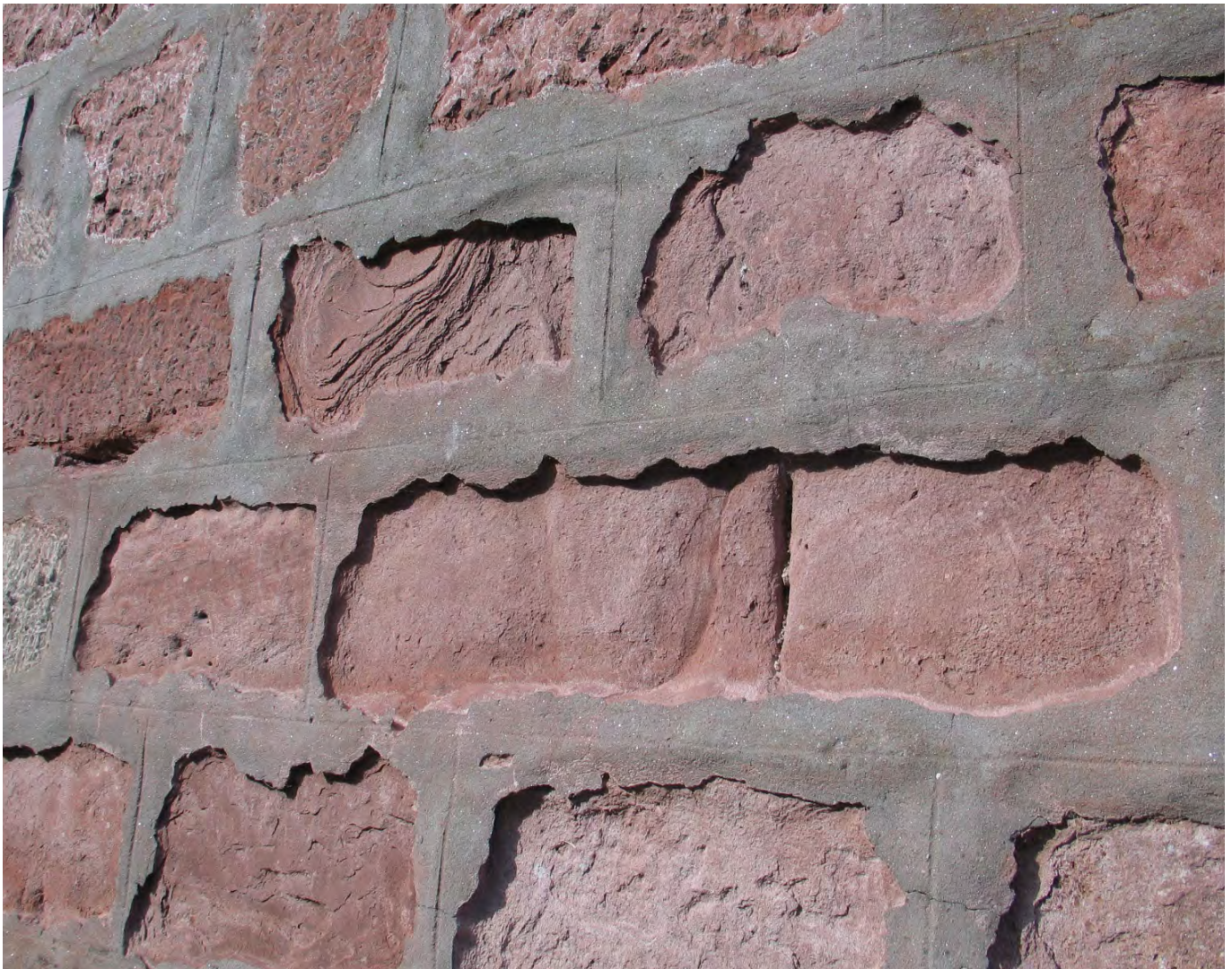
Above: Cement mortar to this stone wall has led to increased stone decay.
