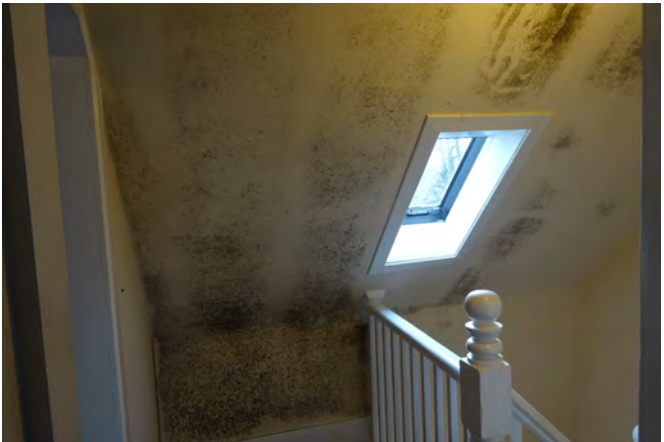
Above: Mould build-up at the top of a staircase, likely due to excess condensation.
