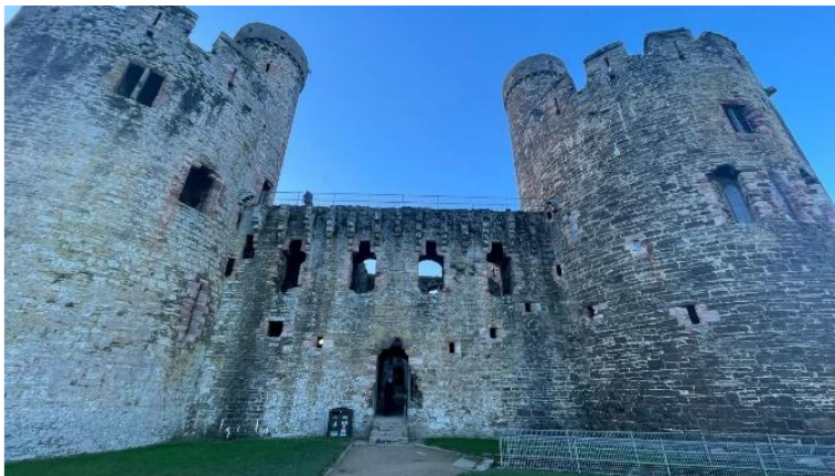
East Barbican at Conwy Castle
