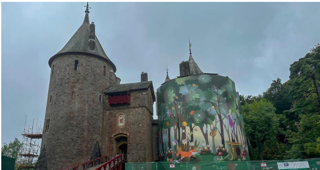
Decorative scaffolding wrap at Castell Coch
