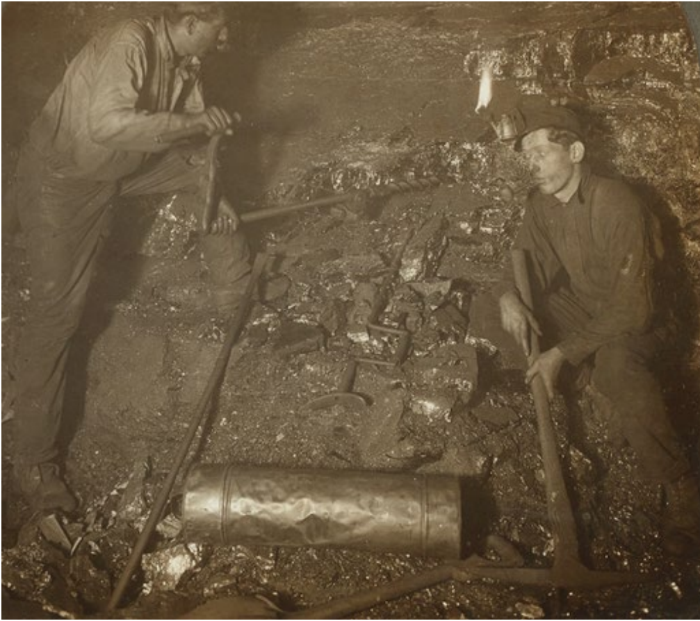
Drilling in preparation for blasting
