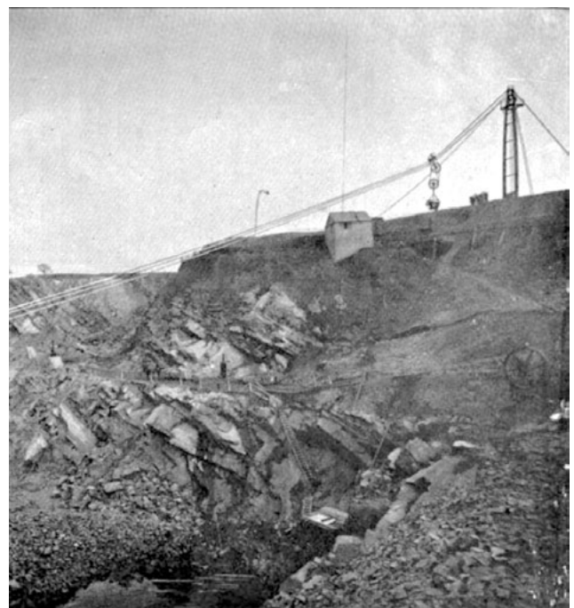
A blondin at Stoney Stanton quarry, showing the cableway crossing a deep pit. Public Domain
