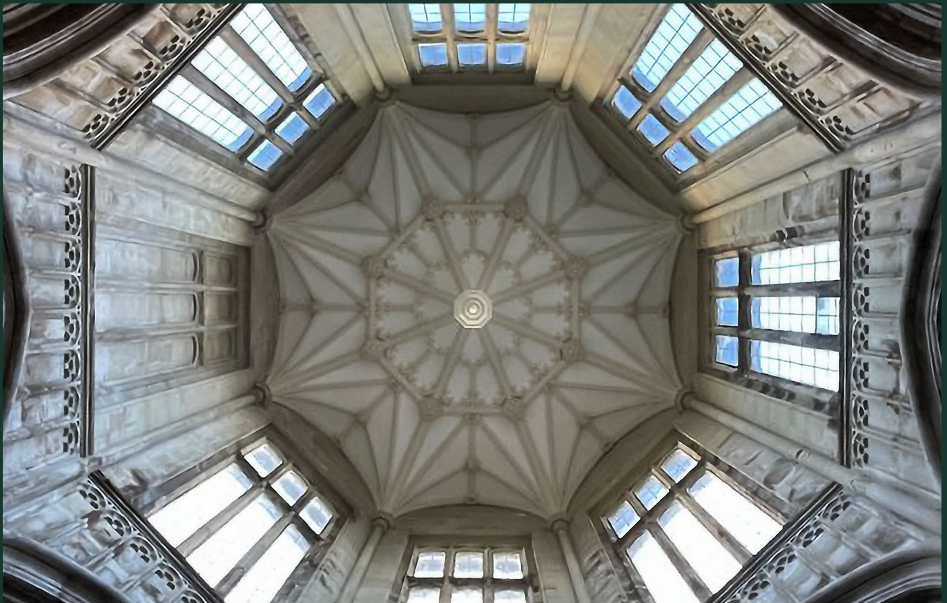
The restoration of Margam Castle's ornate plaster ceiling, supported by Cadw funding, provided hands-on training in traditional stone masonry skills.
